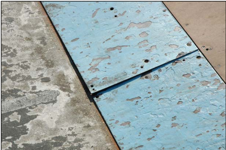
Metal flashing is loose and missing screws on several of the ramps.
