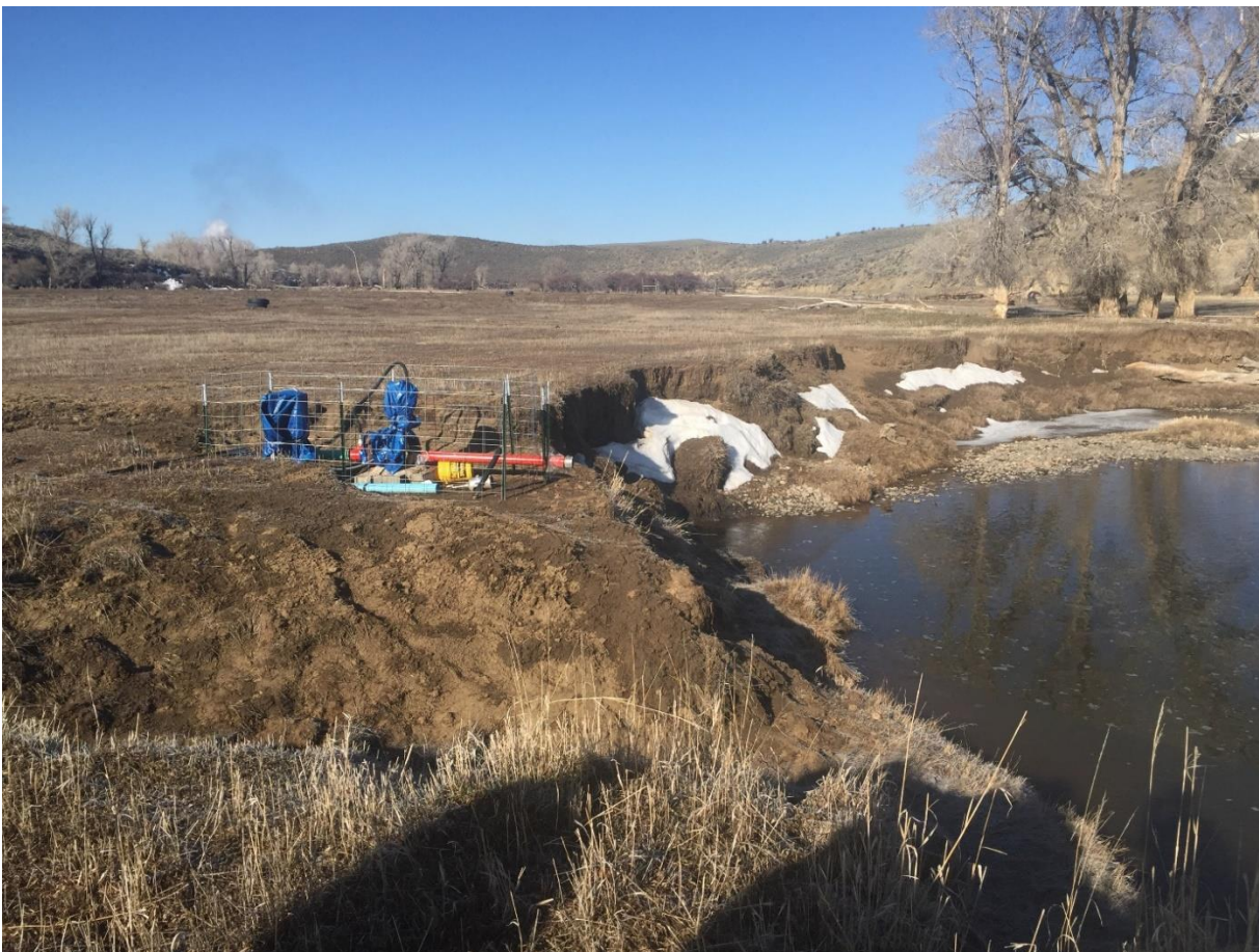
4. Excessive erosion putting existing irrigation infrastructure at risk.
