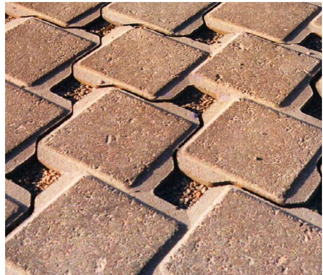
Permeable pavers allow water to filter, thus reducing storm water runoff.
