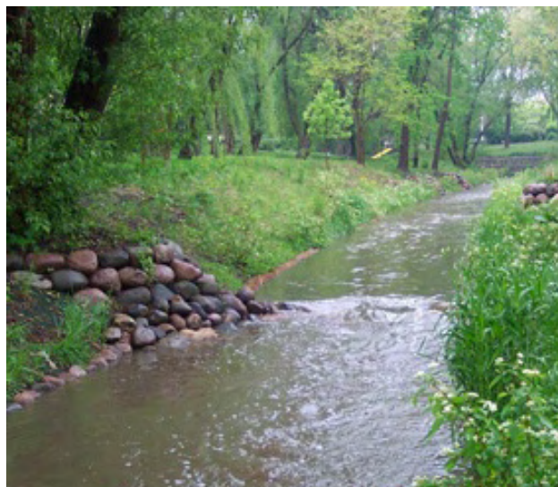
Stream bank stabilization along Salt Creek
