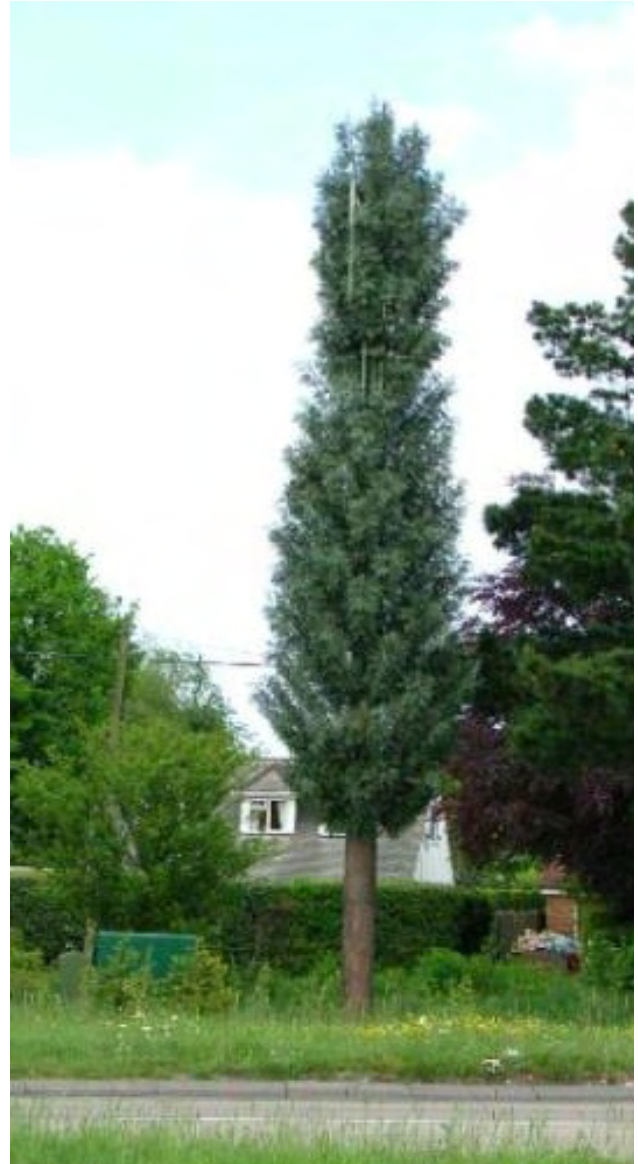
‘Stealth Technology’ in use ; the cell phone tower is disguised
