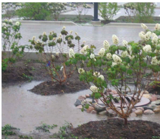
A swale absorbs rainwater, thus reducing storm water runoff.
