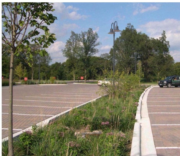
Vegetated Swale reduces impervious surface..
