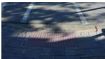
Existing curb ramp with tactile surfaces
