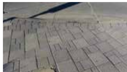
Existing curb ramp without tactile surfaces
