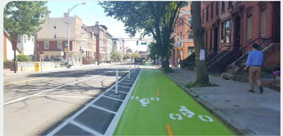
Two-way protected bike lane in Jersey City, NJ; Photo by City of Jersey City
