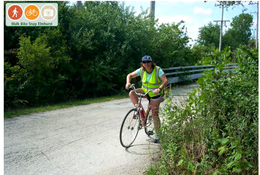
Top Priority: "Because of overgrowth you cannot see bikes or people coming over the IL-83 Bridge on the Prairie Path Trail." Photo by Ted
