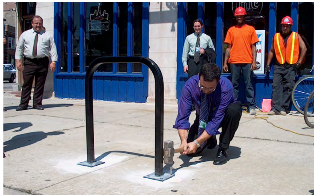
Bike rack installation
