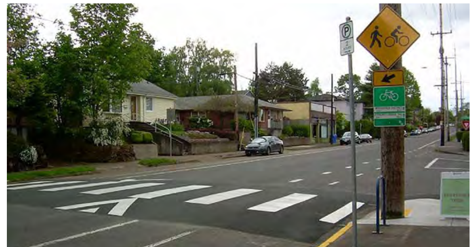
Raised crosswalk image courtesy of FHWA
