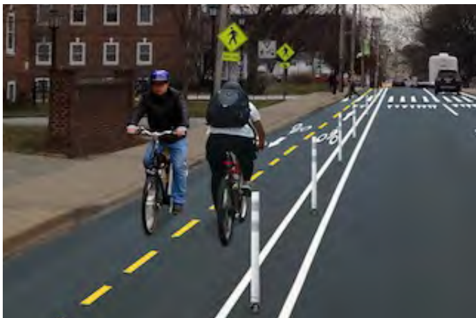
Two-way protected bike lanes with bollards; Photo by Bike Newark
