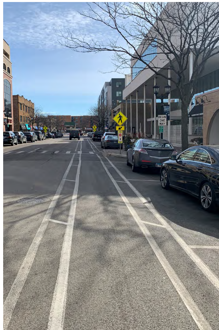
An existing buffered bike lane in downtown Elmhurst on Addison Ave
