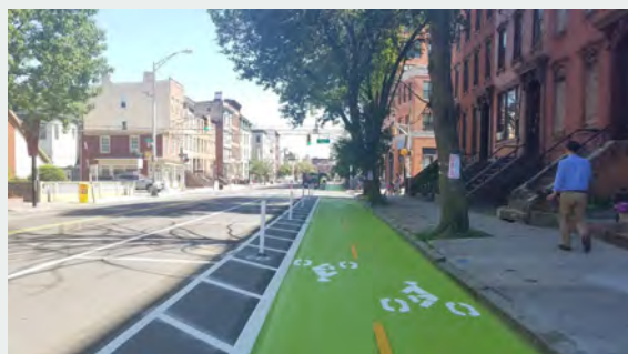
Two-way protected bike lane in Jersey City, NJ; Photo by City of Jersey City
