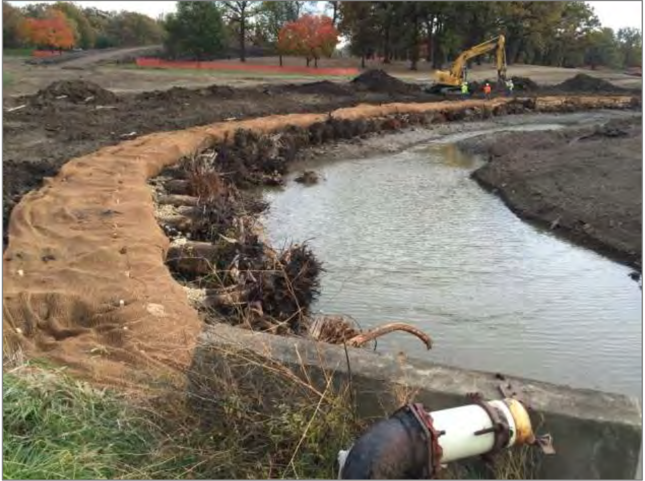
Plate 4. Work in the drained Salt Creek channel showing root wads and bank protection fabrics (image FPDDC).
