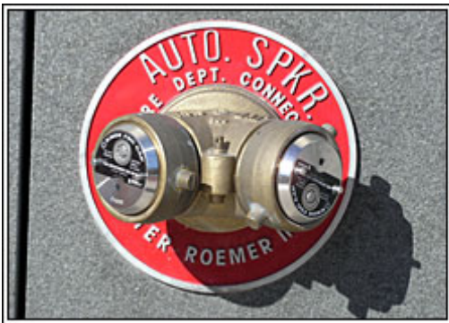
Example of a properly protected FDC
