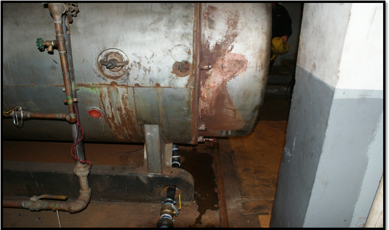
FLHS 1971 boilers showing age, rusting and leaks
