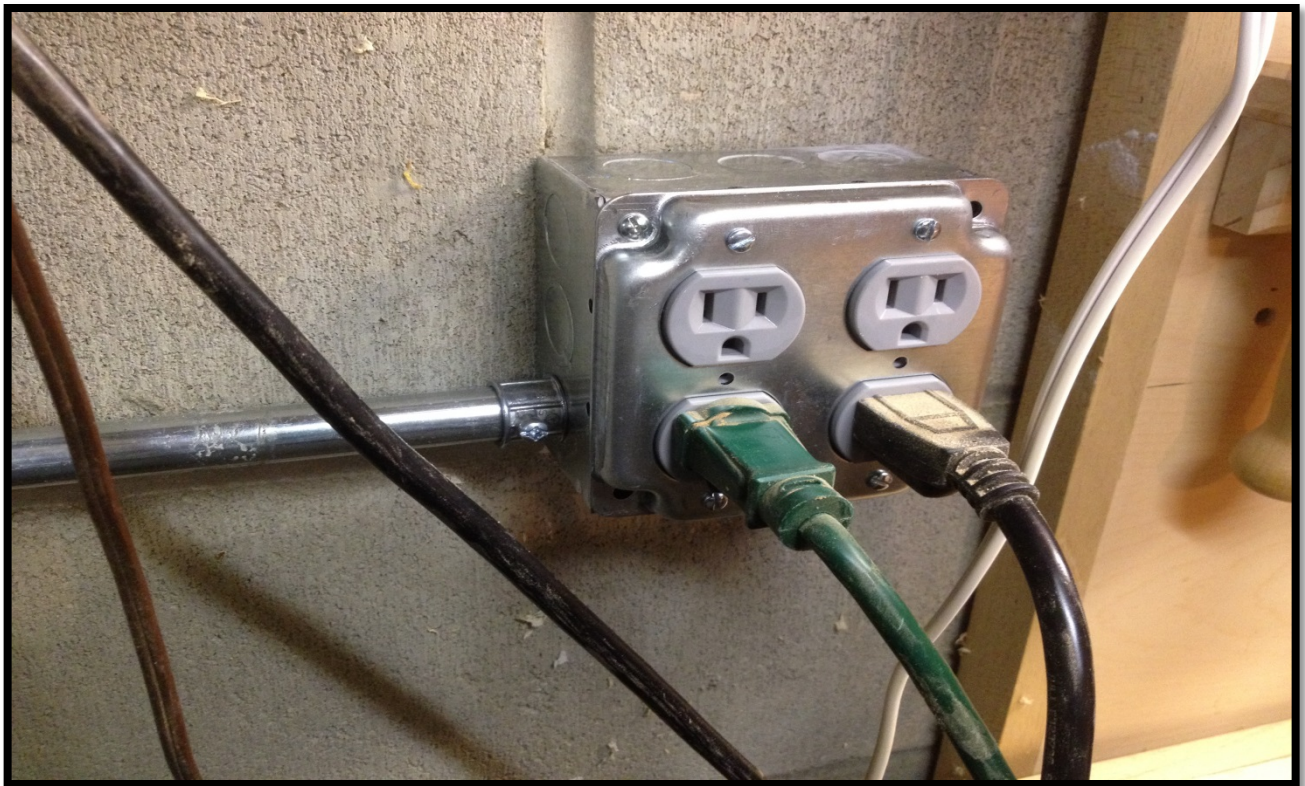
Electrical power quad outlet
