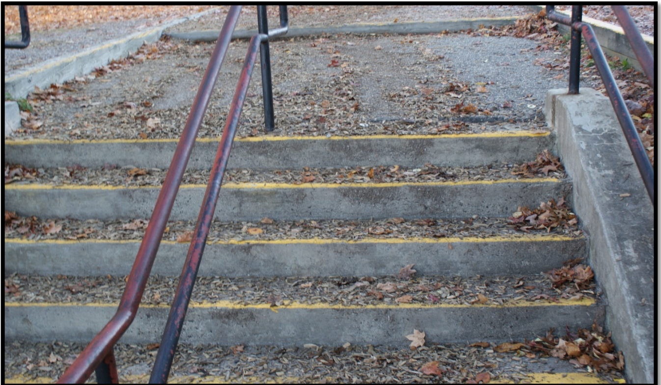
Dwight Elementary School playground wood fiber chips washing down stairs causing unsafe conditions
