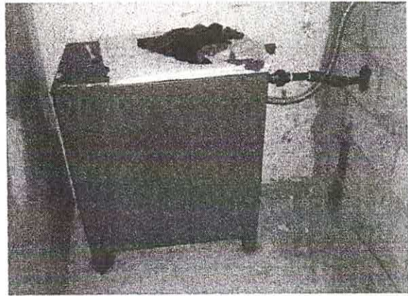
Building 1 elevator hydraulic tank.
