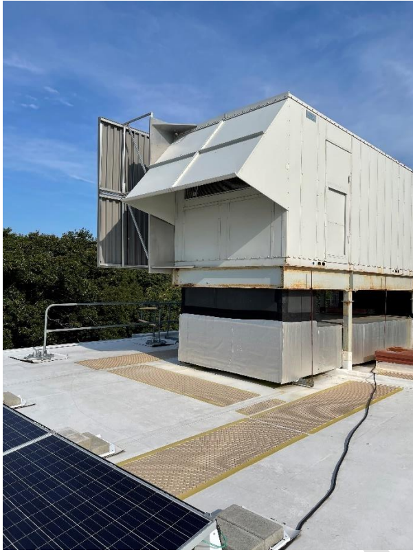
Rooftop Packaged Air-cooled Electric Heat Unit Serving the north wing.
