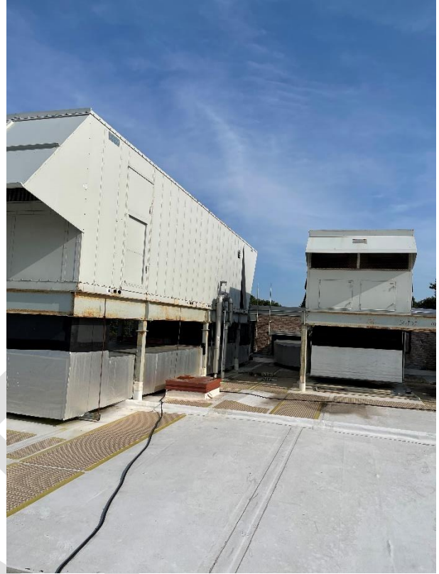
Rooftop Packaged Air-cooled Electric Heat Unit Serving the north wing.
