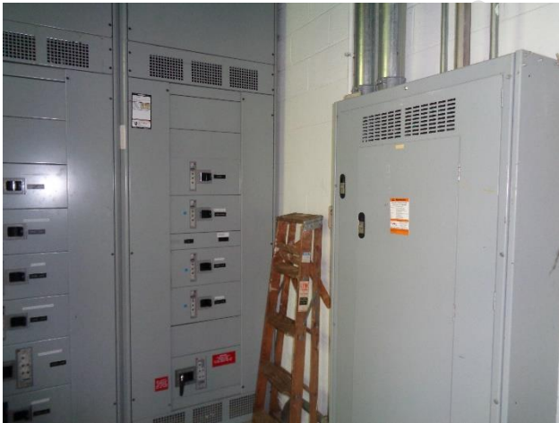
Existing Switchboard
