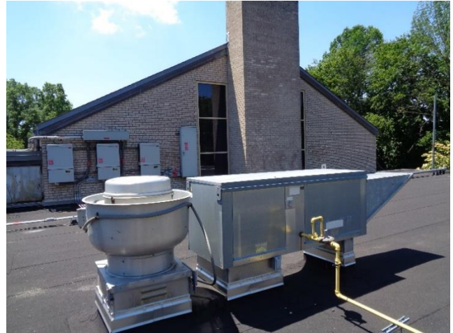
Existing Kitchen Make-up and Exhaust
