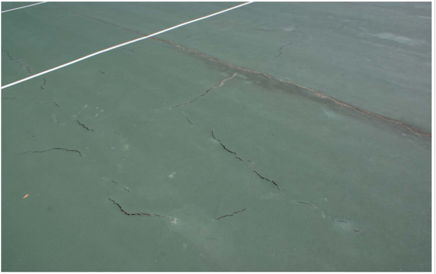
FWHS Blake Tennis Courts showing cracks and uneven surface
