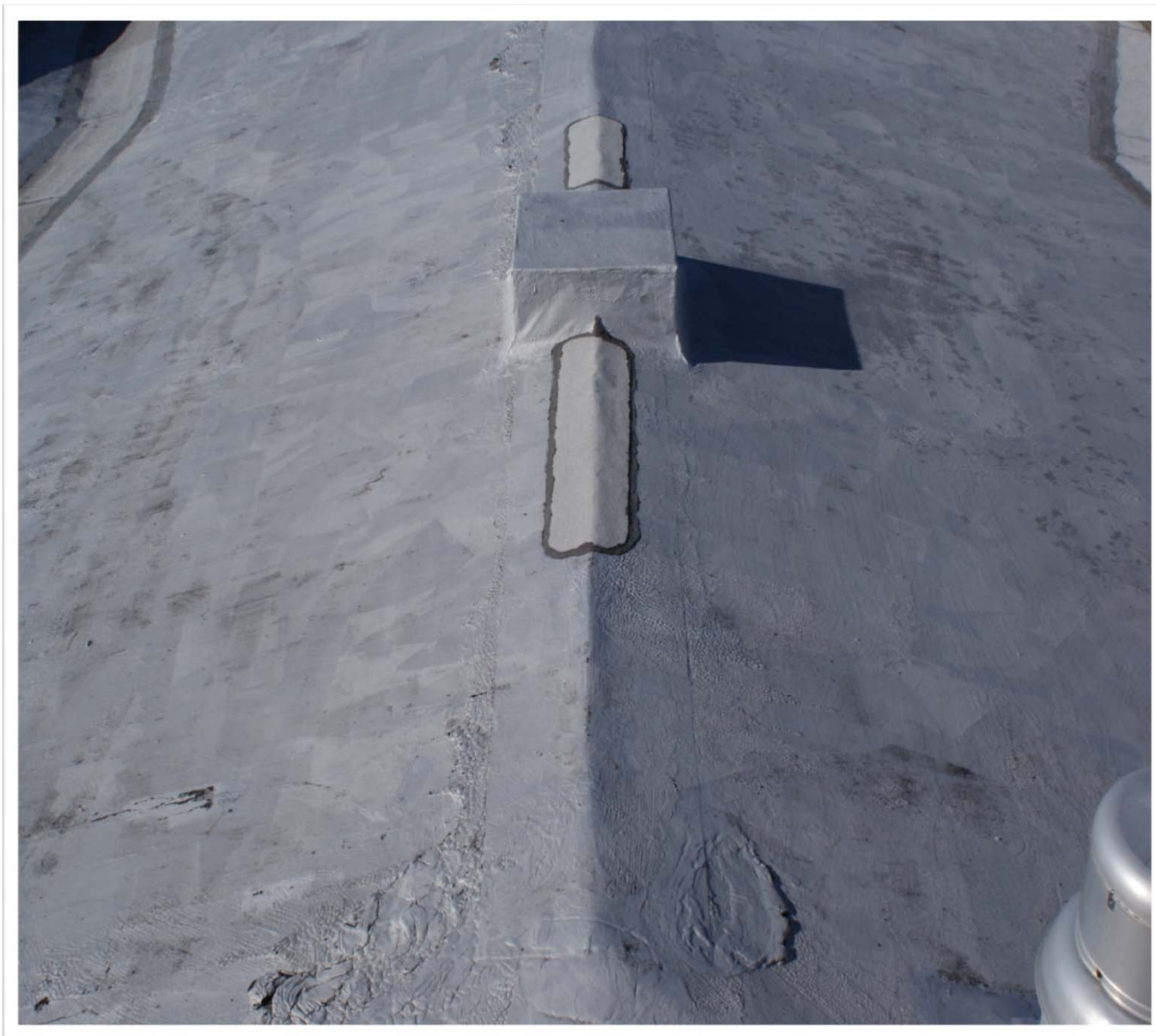
TMS existing roof showing signs of failure and membrane deterioration – warranty expired in 2011
