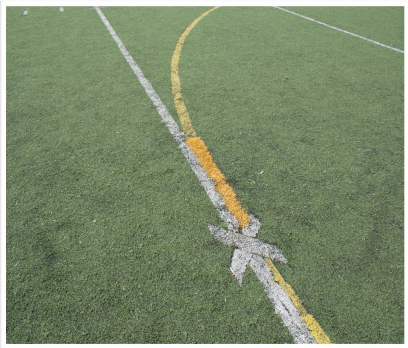
FWHS existing artificial turf field showing deterioration and a patched repair
