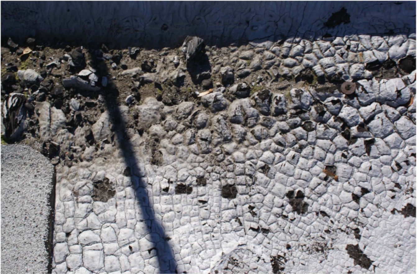
TMS existing roof failures and deterioration up close
