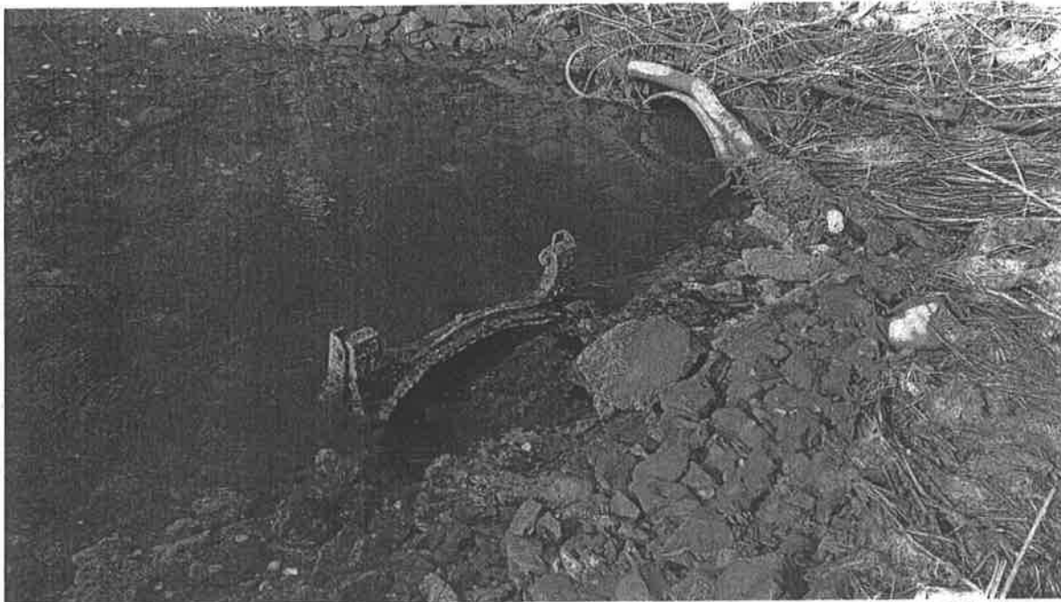
Photo 14: Marina Culvert Entrance Upper Right, South Benson Road Culvert Collapse Center
