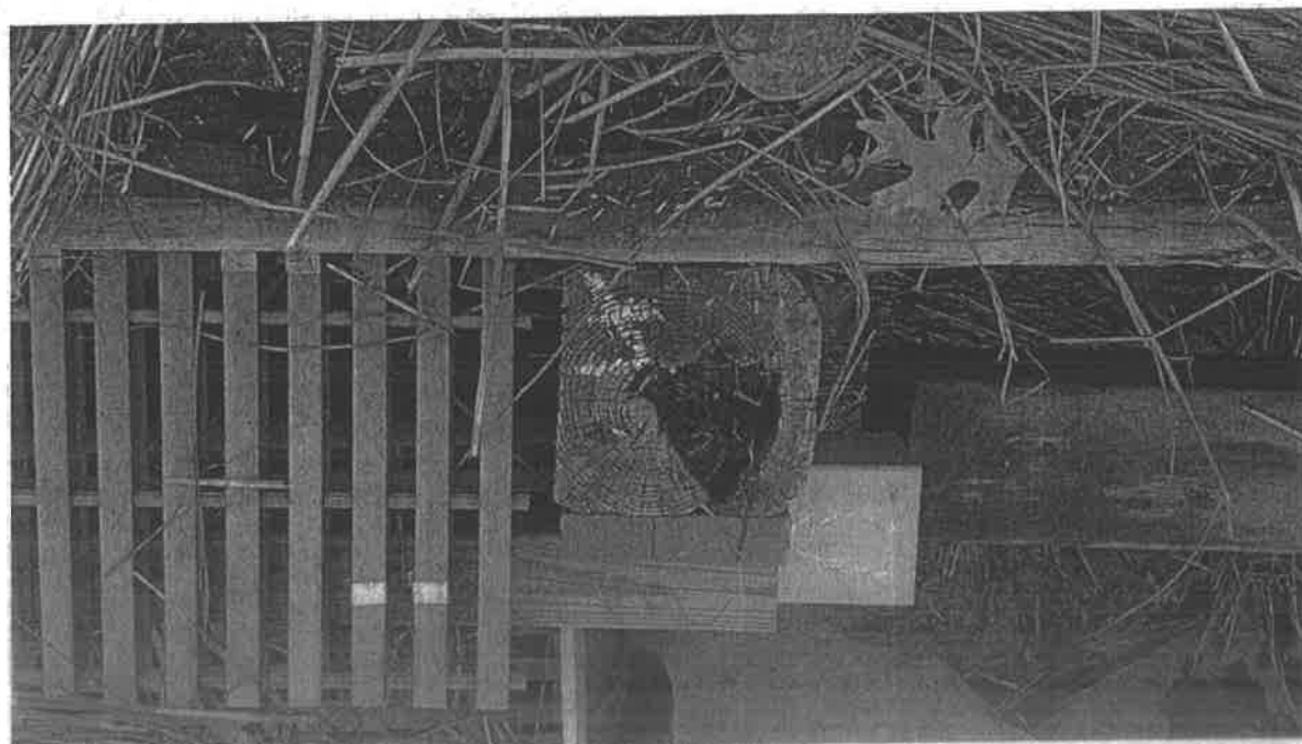
Photo 16: Timber Wall With Decay at Tide Gates
