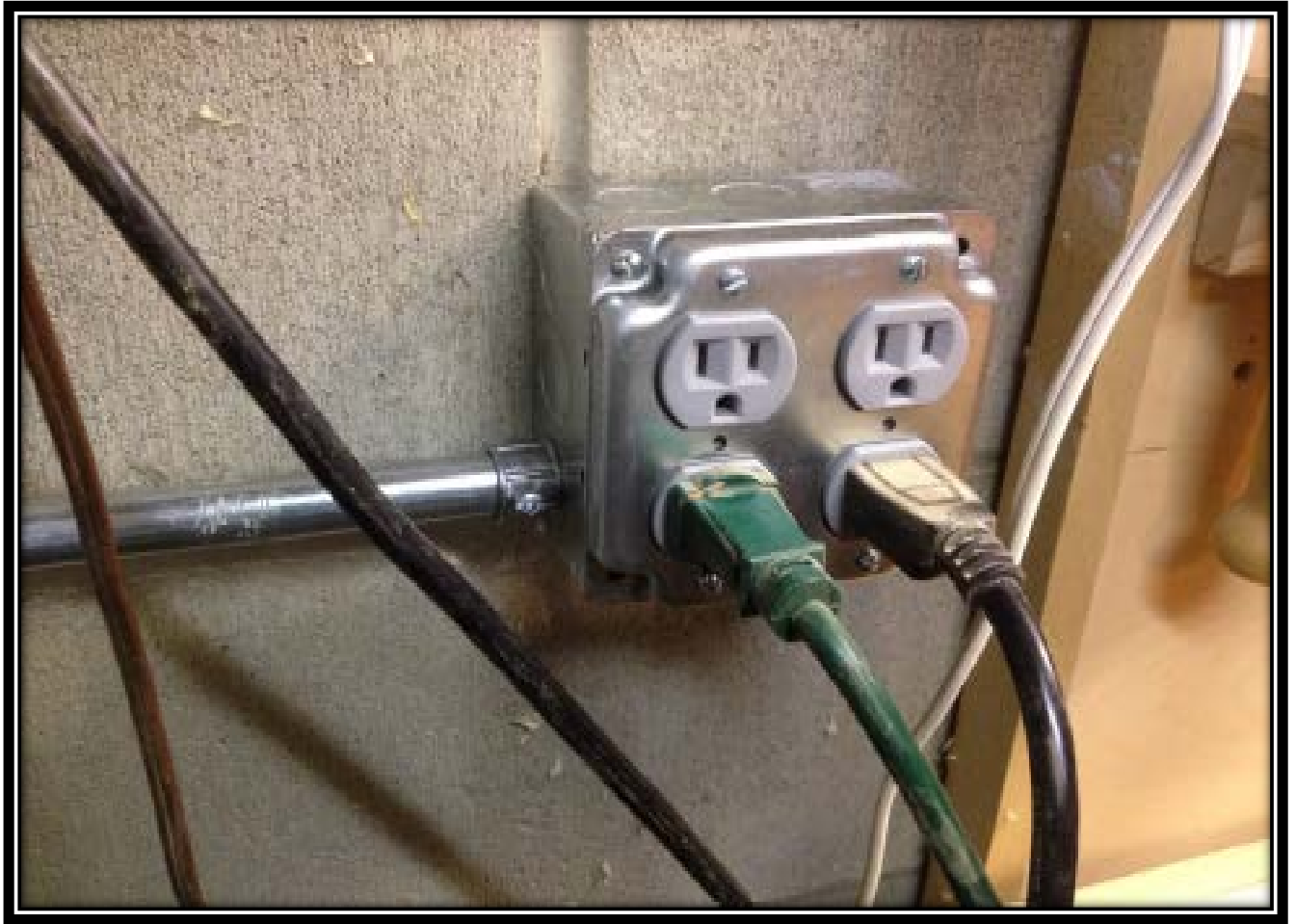
Electrical power quad outlet
