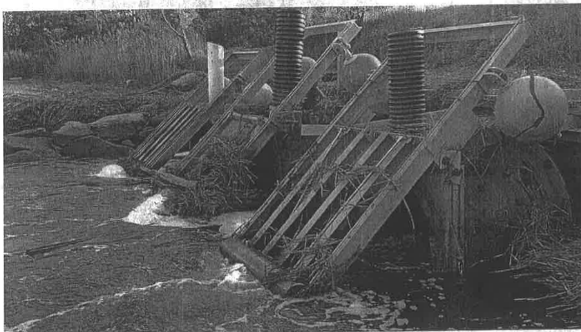
Photo 15: Overview of Tide Gates - Center Gate is Fiberglass
