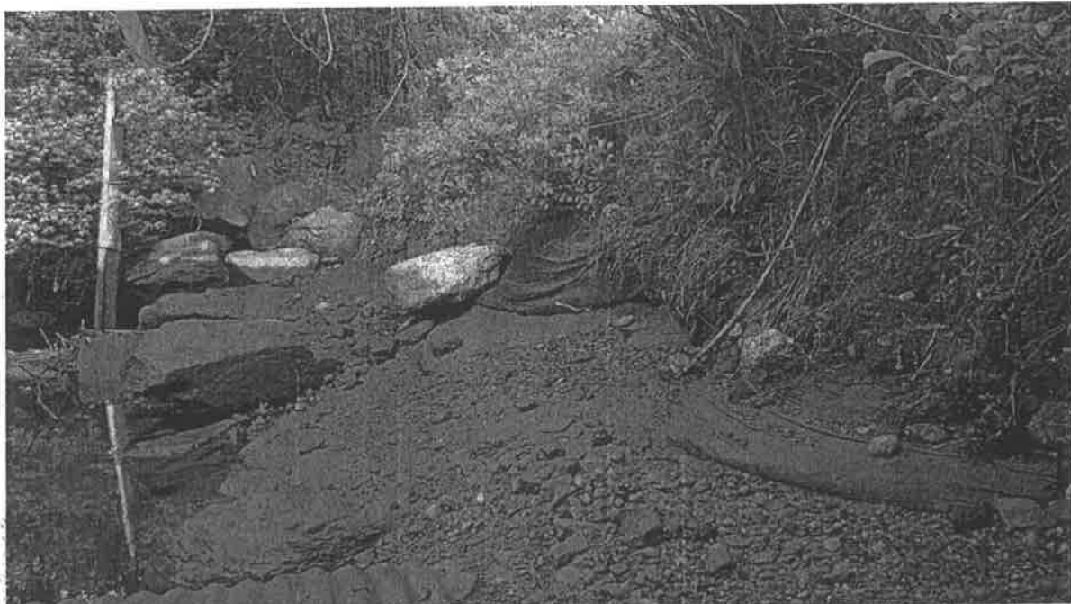
Photo 18: Tide Zone Bank Erosion with Exposed Geotextile
