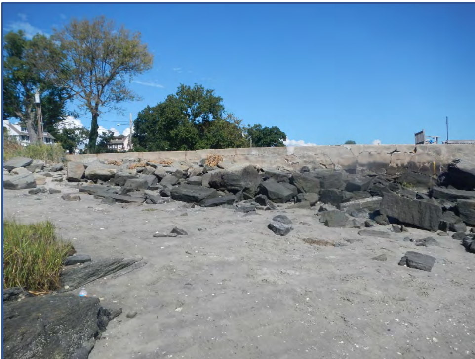
Photograph 4: Existing Beach and Stone Revetment Along Seawall
