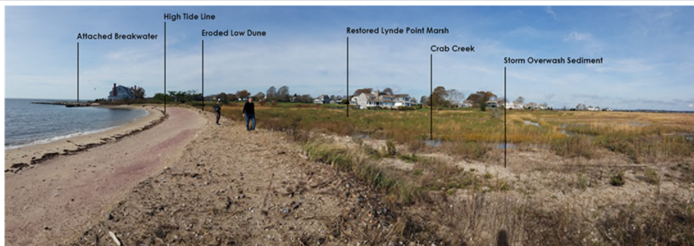
A view of the existing Hepburn dune, barrier spit beach and tidal marsh, Fenwick, CT. The dune is almost completely eroded, and the remaining beach is narrow.
