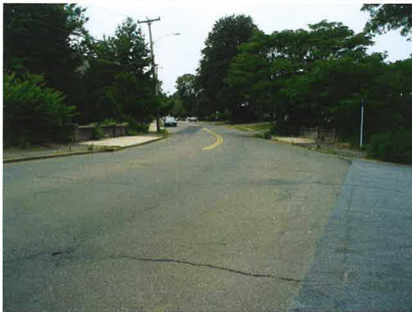
Photo # 1: View of East Approach. Notice Cracking of Approach Roadway.
