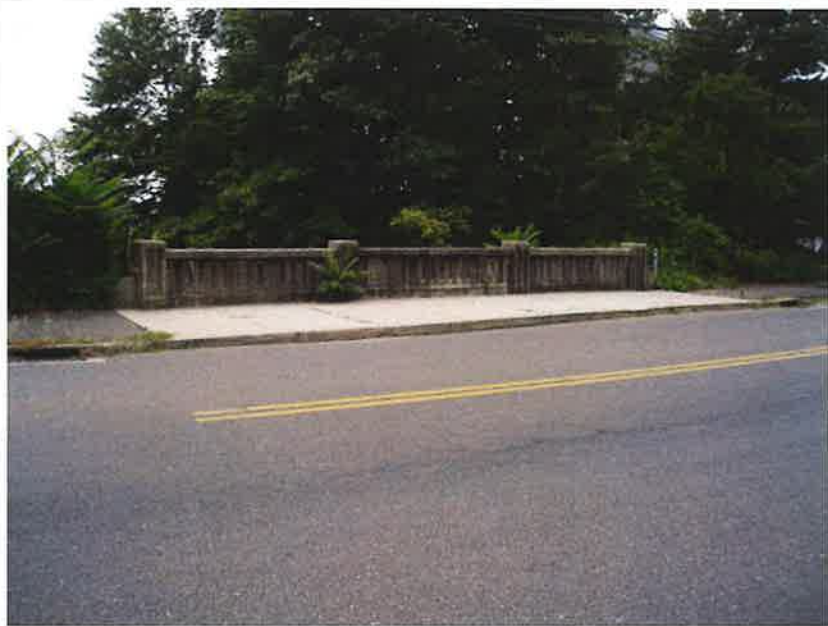
Photo # 2 View of South Parapet Wall. Notice Minor Cracking of Bituminous Wearing Surface.
