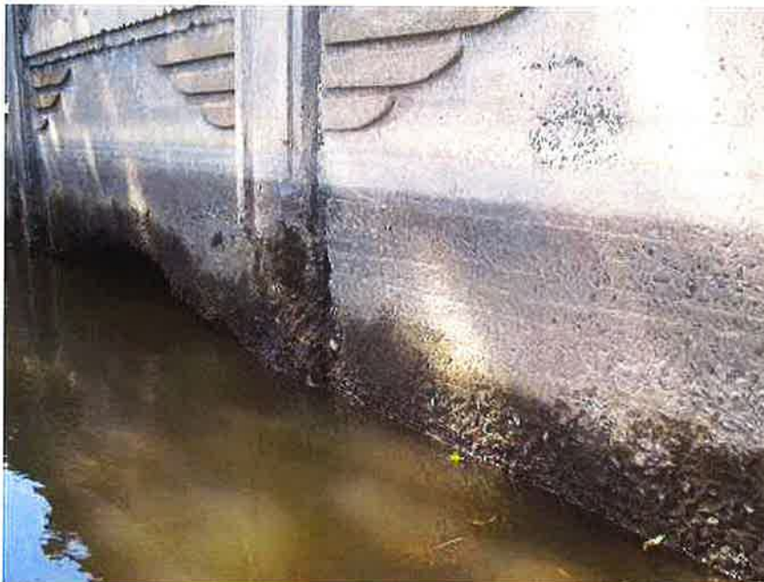
Heavy scaling along edge of opening extending into wingwalls below waterline at outlet.
