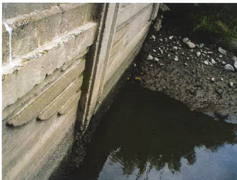
Photo # 7: View of Southeast Embankment. Notice Spalled Concrete at Water Level.
