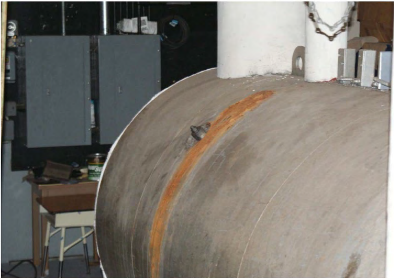
Old 1966 boilers showing age and leaks
