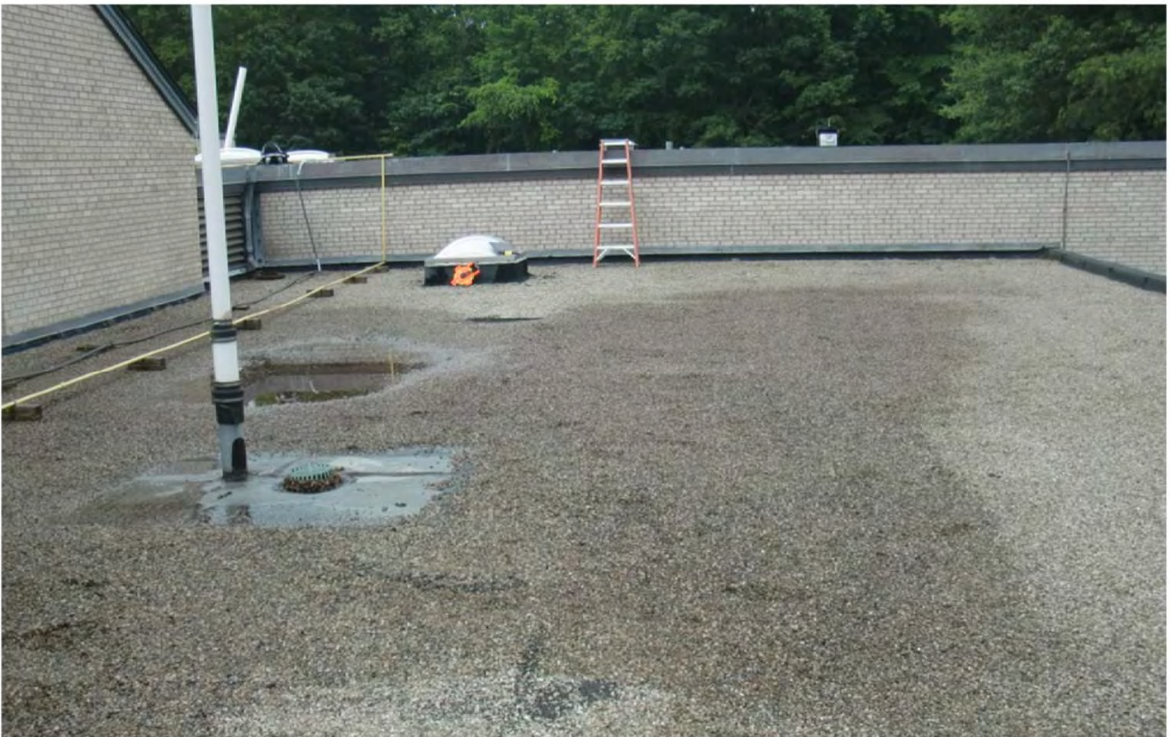
More roof patches and ponding of water failures
