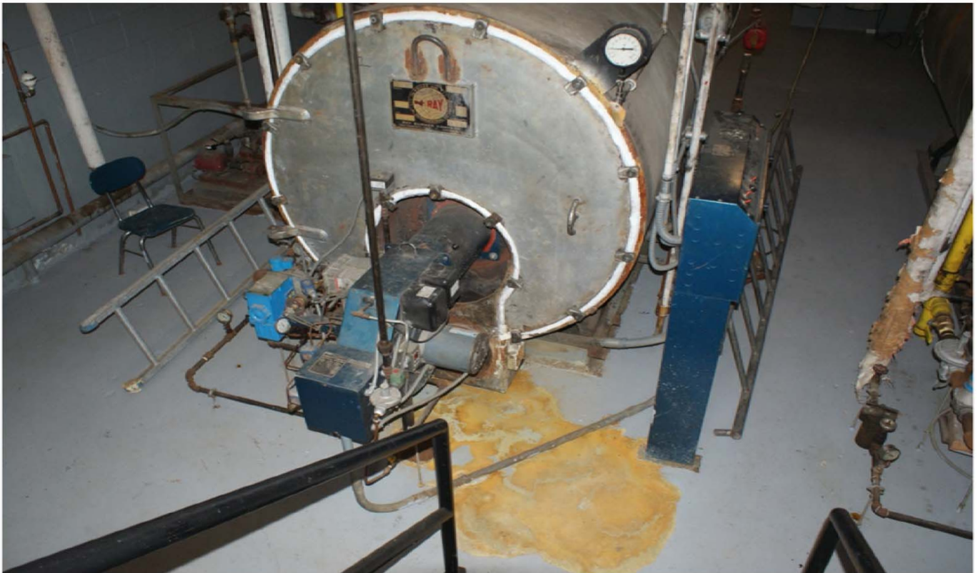
Old 1966 boilers showing age and leaks
