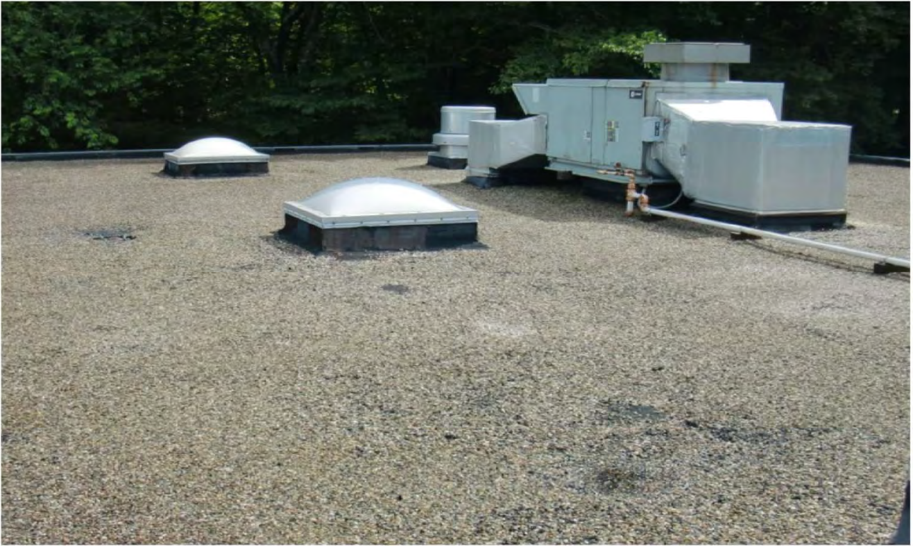
Old roof membrane failures and patches around skylight
