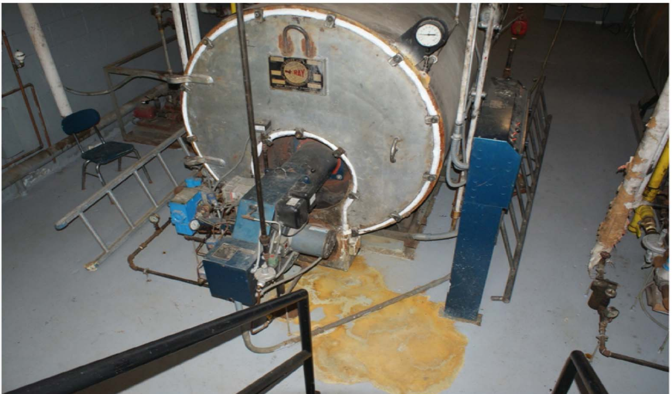
Old 1966 boilers showing age and leaks
