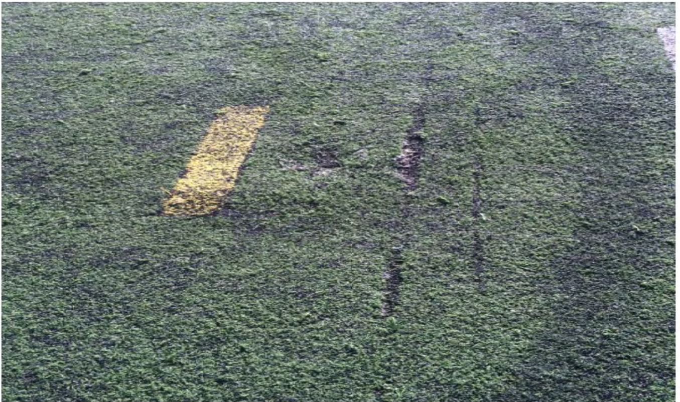
Close up field deterioration
