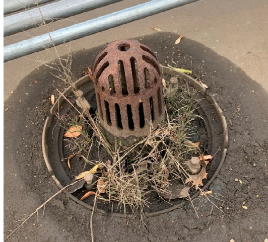
Example of outdated and ineffective roof drain grate
