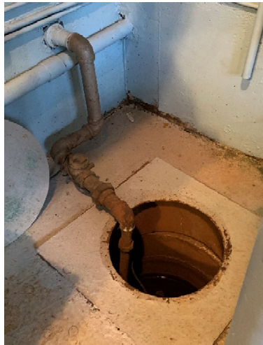
Existing Sump Pit in Boiler Room
