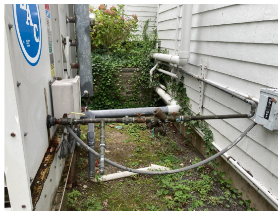
Exterior Cold-Water Piping to the Cooling Tower
