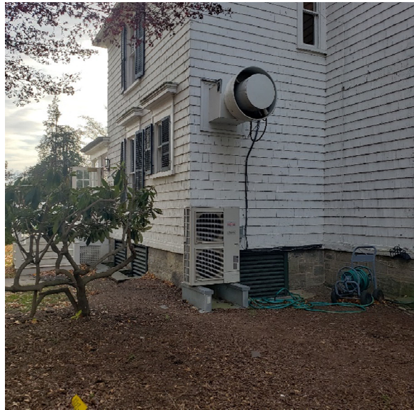
Existing kitchen exhaust fan & outdoor heat pump.
