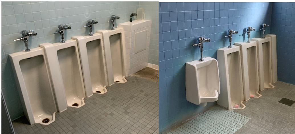
Examples of Existing Urinal Fixtures
