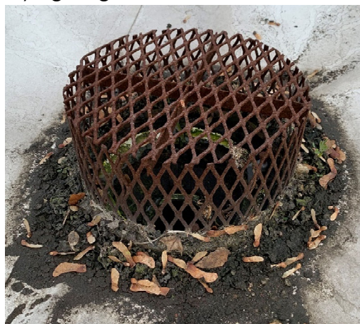
Example of outdated roof drain grate
