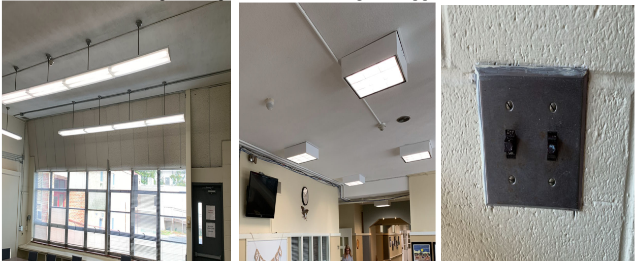
Bigelow Light Fixtures and Original Toggle Switches
