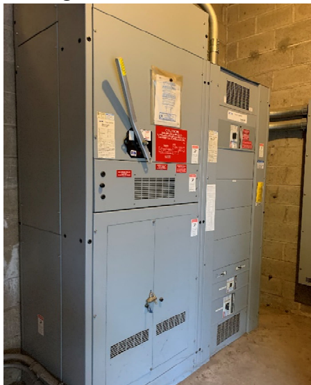
Switchgear and Main Distribution
