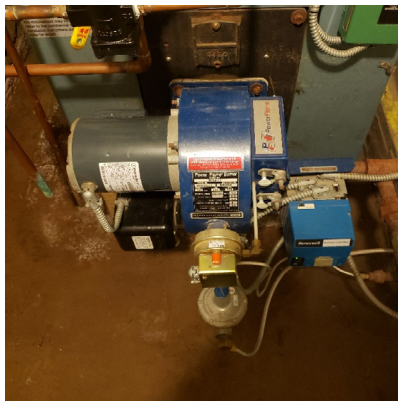
Existing boiler burner
