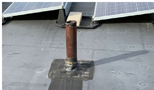
Vent to Roof showing signs of rust
