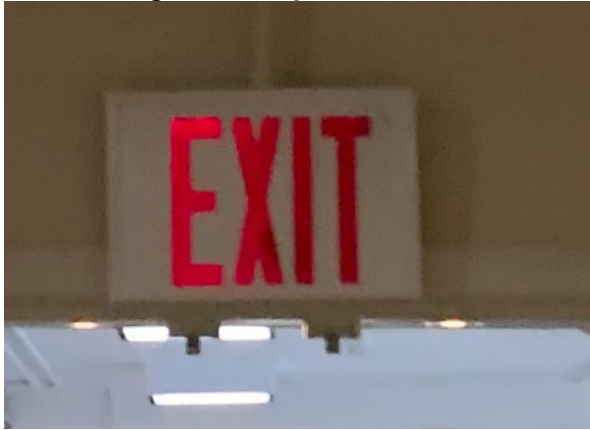
Exit Sign not Fully Illuminated
