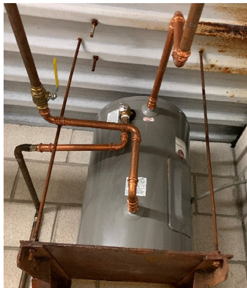
Existing Rheem Electric Water Heater
