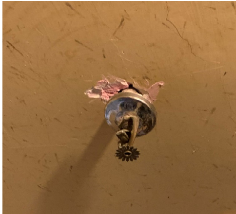
Typical Pendent Sprinkler Head
