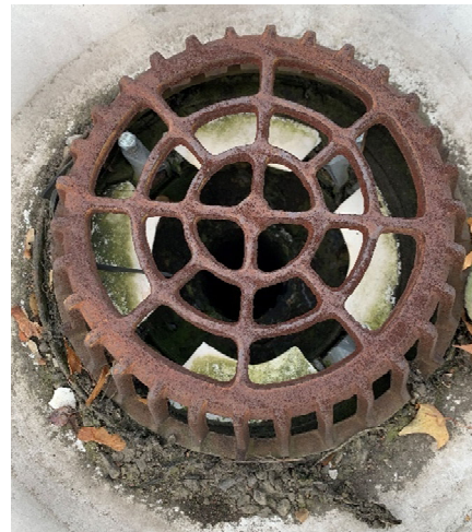
Comparison of varying degrees of wear and tear on roof drain grates
