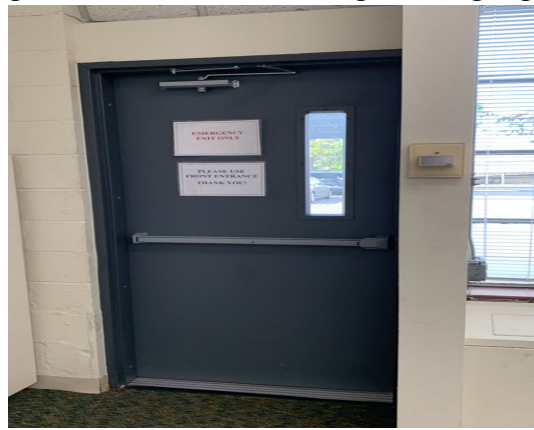
Egress Door without Exit Sign & Emg. Lgt.
