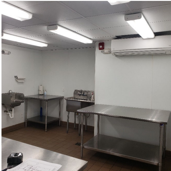
Existing kitchen wall mounted indoor heating/cooling unit
