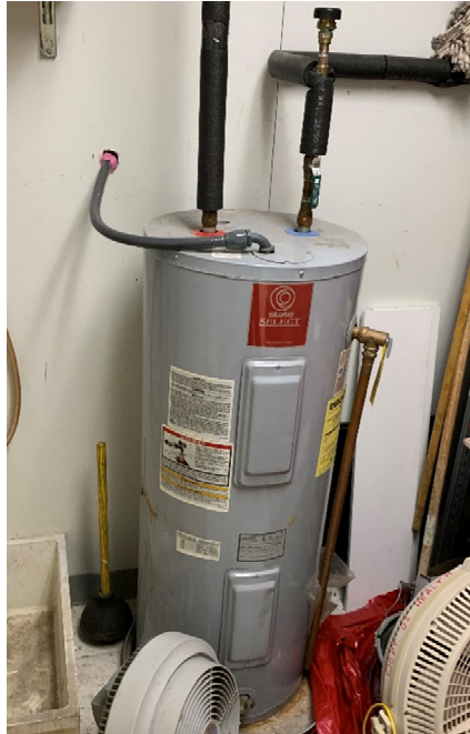
Existing State Industries Electric Water Heater
