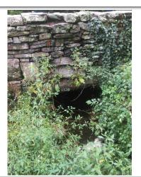
Verna Hill: this culvert had a (CMP PIPE) that was 22'L x 36"D this pipe was completely destroyed due to hydraulic pressure change from WDR
