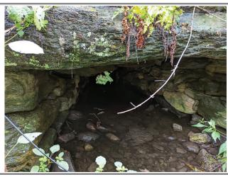
Verna Hill: scouring to head wall and inside of culvert and as a
