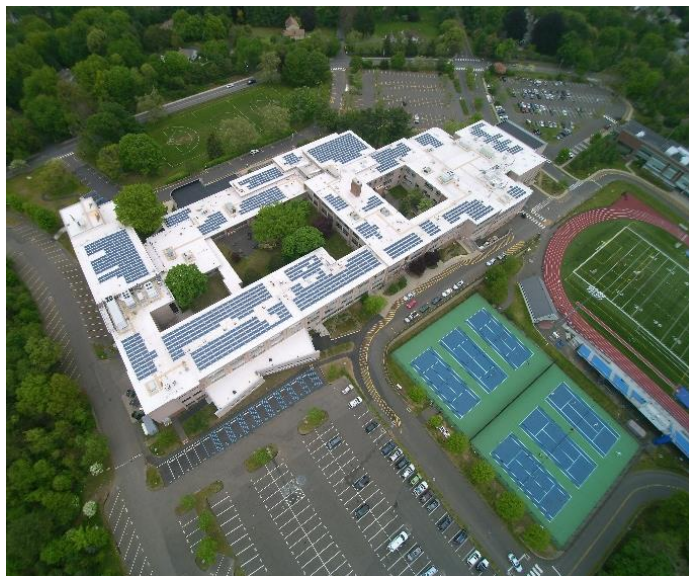
Reflective White Roof and Rooftop Solar Array at Fairfield Ludlowe High School
