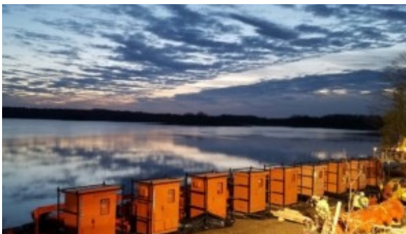
Great Hill Tunnel Pipeline Restoration
