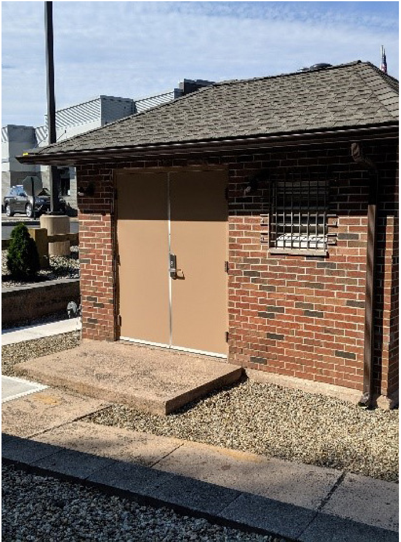
South End Road Pump Station Upgrade, Southington, CT
