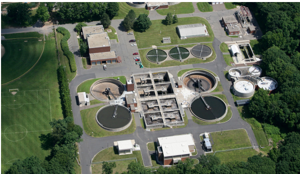
Southington Water Pollution Control Facility Design and Engineering Improvements
