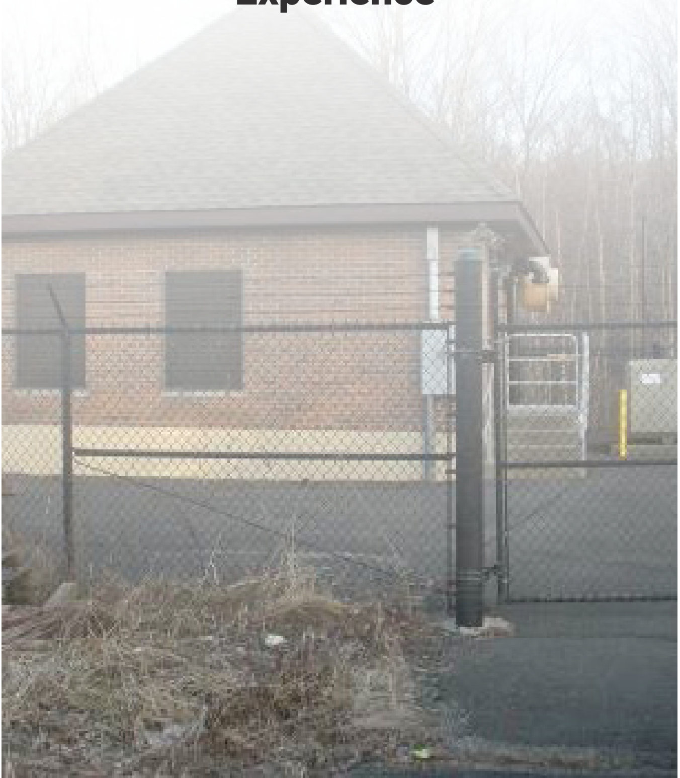
Puimp Station Upgrades, Southington, CTT
