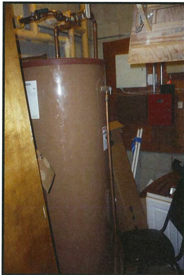
Photo #10: Domestic Hot Water Heater
