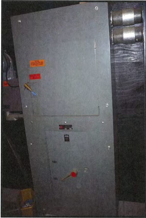
Photo #13: Main Switch & Metering Compartment
