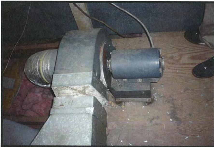
Photo #6: Bathroom Exhaust Fan
