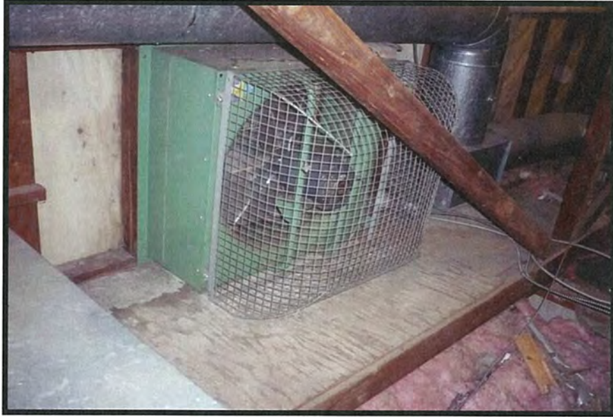
Photo #5: Attic Exhaust Fan
