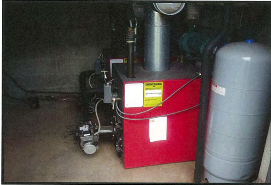
Photo #1: Oil Fired Boilers
