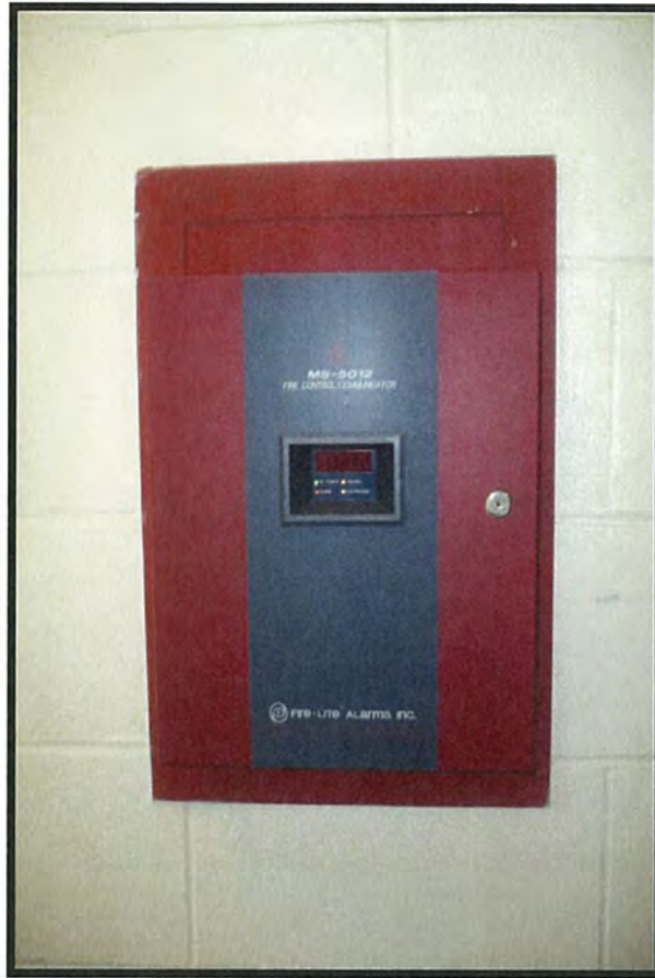
Photo #11: Fire Alarm Panel
