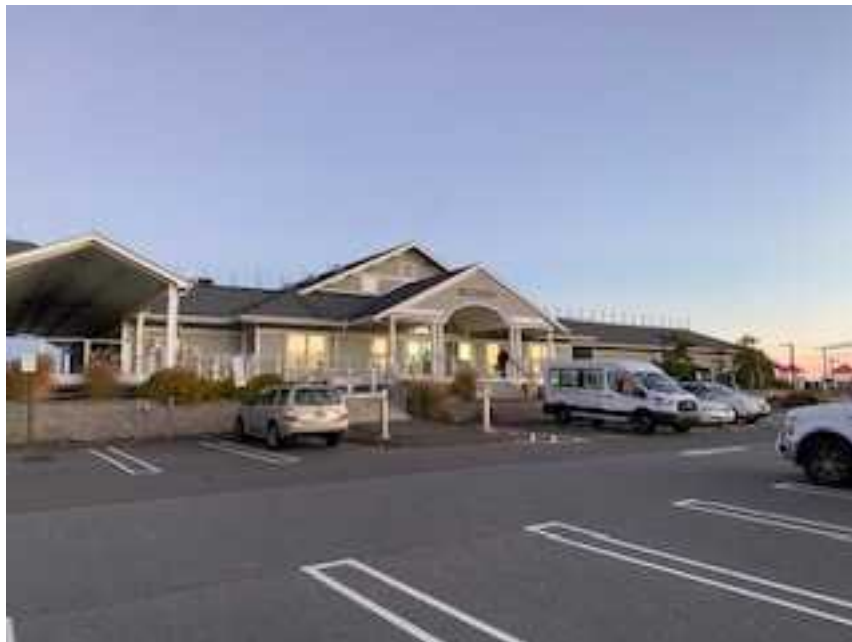
FRONT AND SIDE VIEW OF BUILDING LOOKING SOUTHWEST
