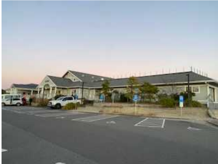
FRONT AND SIDE VIEW OF BUILDING
