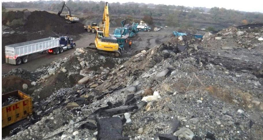
Long-stick excavator in background atop large pile of screened material. The soil is being loaded into trucks for offsite use. In foreground, Komatsu excavator is loading material from the southern end of the main pile into the screener.
