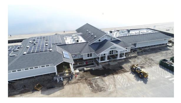
Significant progress has been made by our contracted construction team at the Penfield Pavilion. The demolition phase of the decks, ramps and stairs is nearing completion. The contractor is now preparing to commence excavation work around and under the building. Excavation around the building will facilitate various aspects of the job including access to below the building to allow for grade beam demolition.
