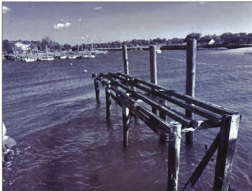
Photograph 23 - Remaining timber wharf T-head
