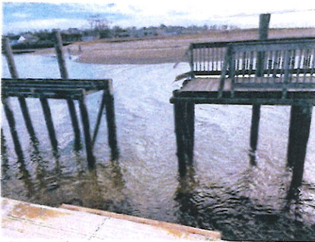
Damaged Pier from recent storm
