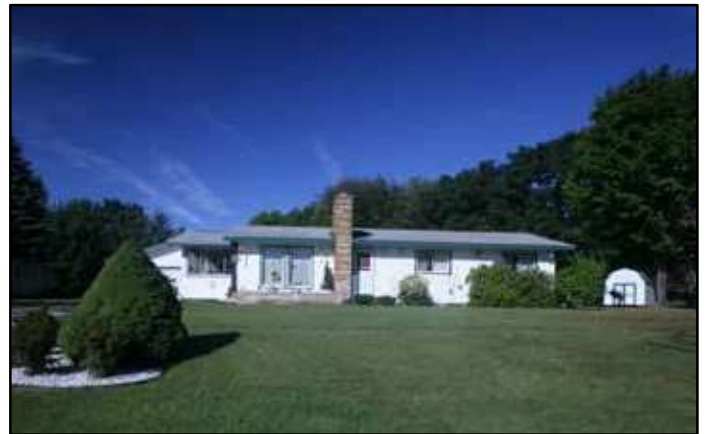
Example of non-historic architecture common in the East City Residential District. (photo: William Allin Storrer)
