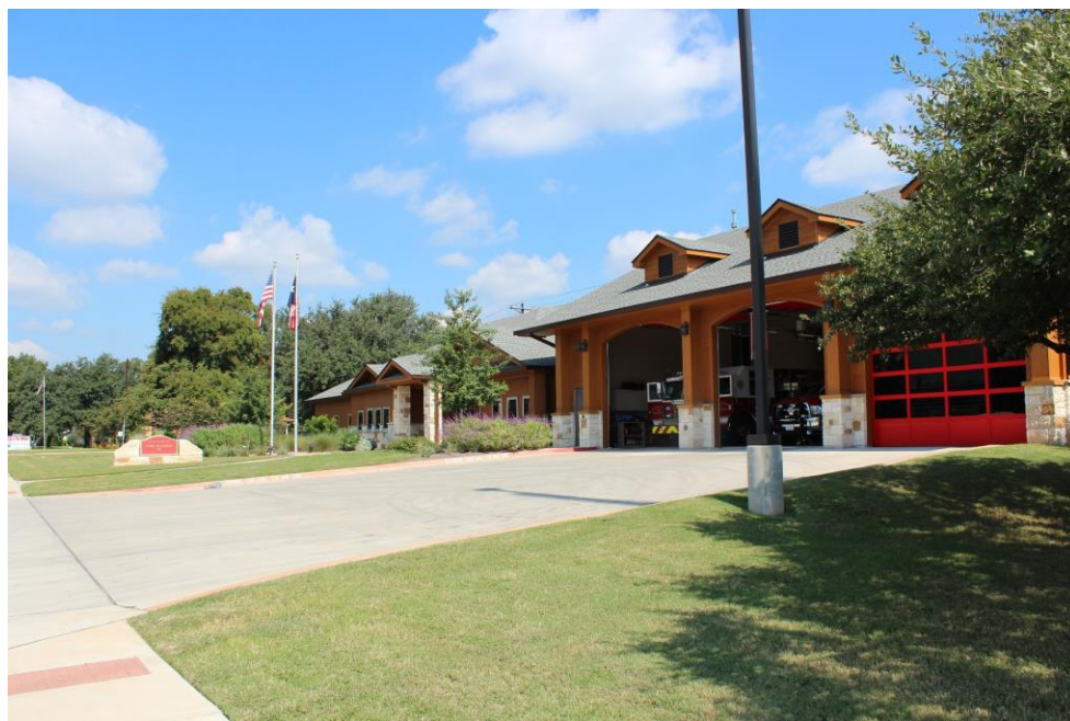
Figure 48. Public Use on Williams Drive
