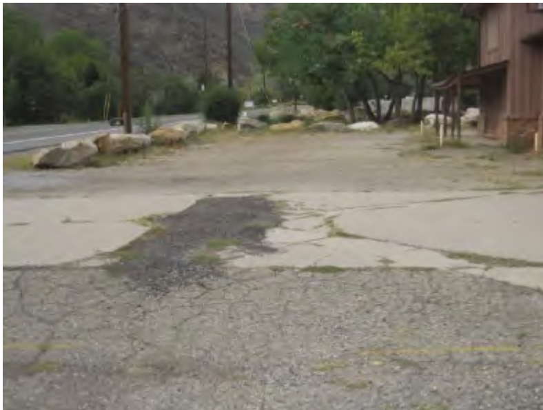
Figure 2-2: Deteriorated pavement, poor parking lot layout, lack of outdoor lighting
