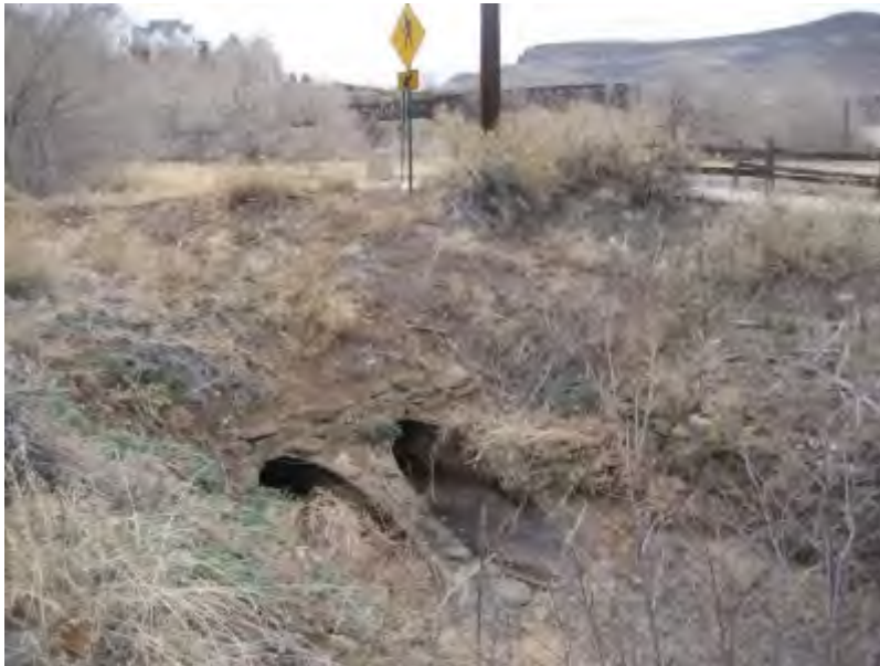
Figure 2-9: Lack of fall protection
