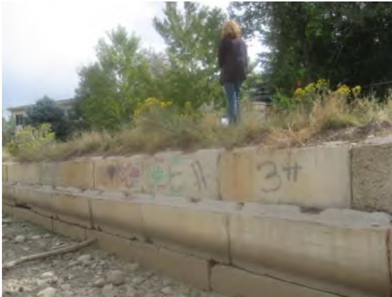
Figure 2-5: Vandalism, lack of fall protection
