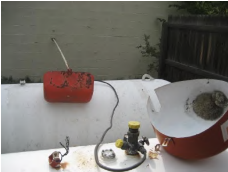
Figure 2-6: Unprotected gas lines and valves
