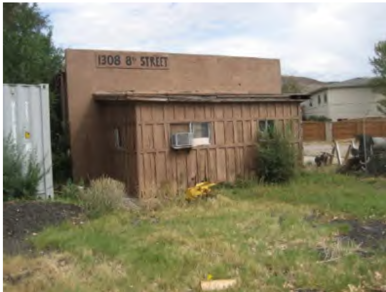
Figure 2-3: Deterioration external surfaces, lack of foundation, lack of gutters/downspouts
