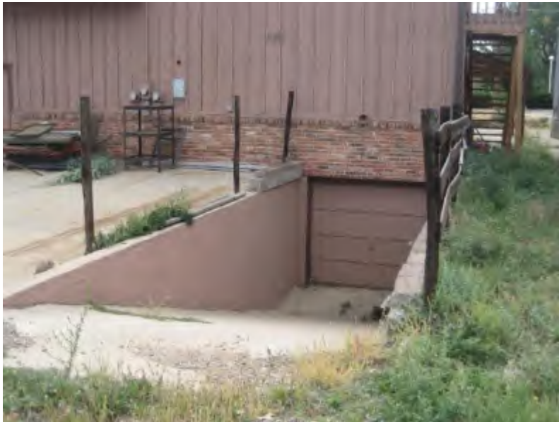
Figure 2-1: Substandard vehicle ramp, lack of fall protection
