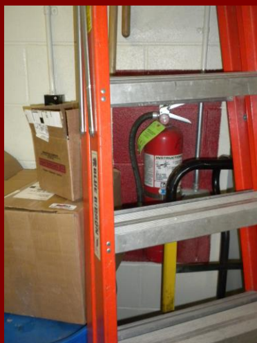
Obstructed fire extinguisher
