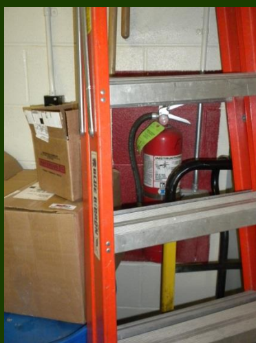
Obstructed fire extinguisher
