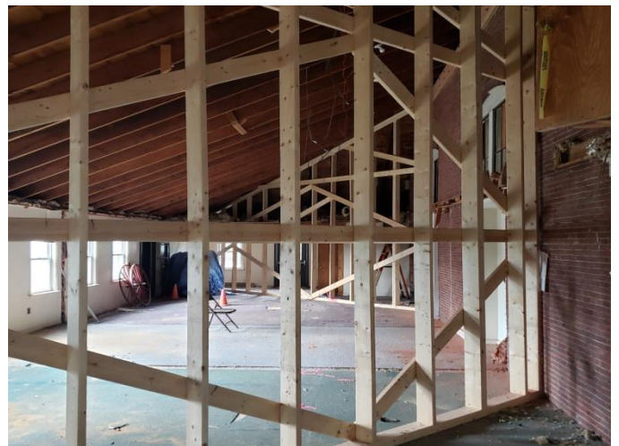
FIGURE 4 PRESENT DAY VIEW OF THE ADDITION SPACE. SUPPORT STRUTS AND A LEDGER BEAM WERE INSERTED IN THE ADDITION SPACE AS AN EMERGENCY PRECAUTION AGAINST SNOW LOADS IN FALL 2018. TAKEN FACING STREET SIDE.
