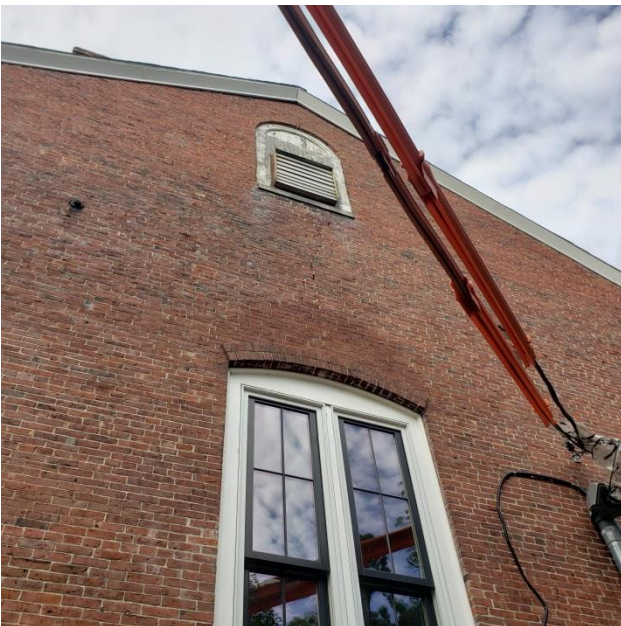
FIGURE 3 EXTERIOR REAR OF THE BUILDING. NOTE A LARGE CRACK IN THE MASONRY BENEATH THE UPPER WINDOW. STAFF WILL MONITOR THE PROPERTY FOR EMERGENCIES, BUT WEATHERING DOES CONTINUE TO AFFECT THE EXTERIOR. THE LONGER THAT THE BUILDING REMAINS UNTREATED, THE COSTLIER TREATMENTS WILL BECOME.
