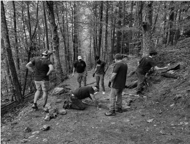
Water bar installation
