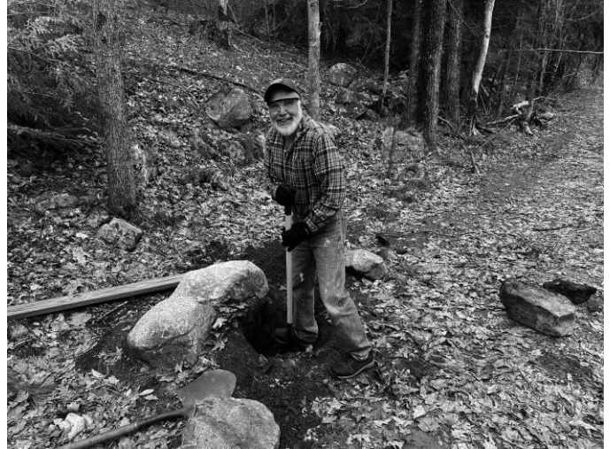
John Pieroni digs a hole for the gate post
