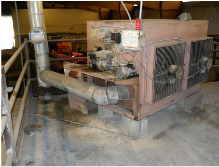
Figure 2. Waste oil furnace
