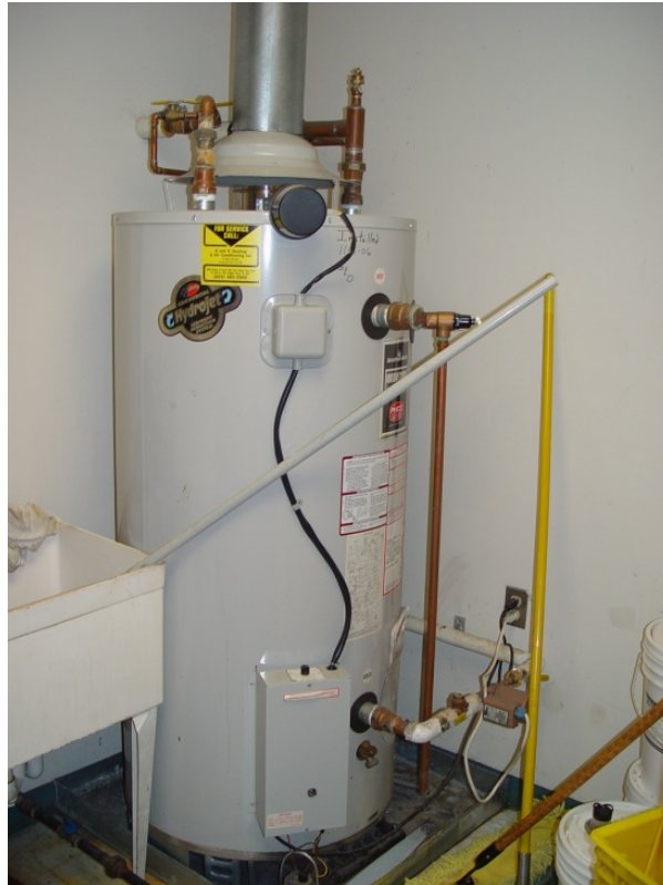
Figure 14. Gas water heater with automatic vent damper
