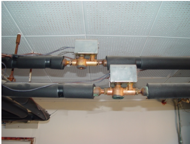
Figure 7. Heating system zone valves
