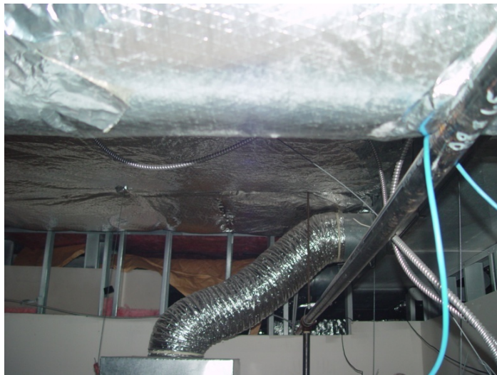
Figure 13. Condition of insulation above ceiling panels
