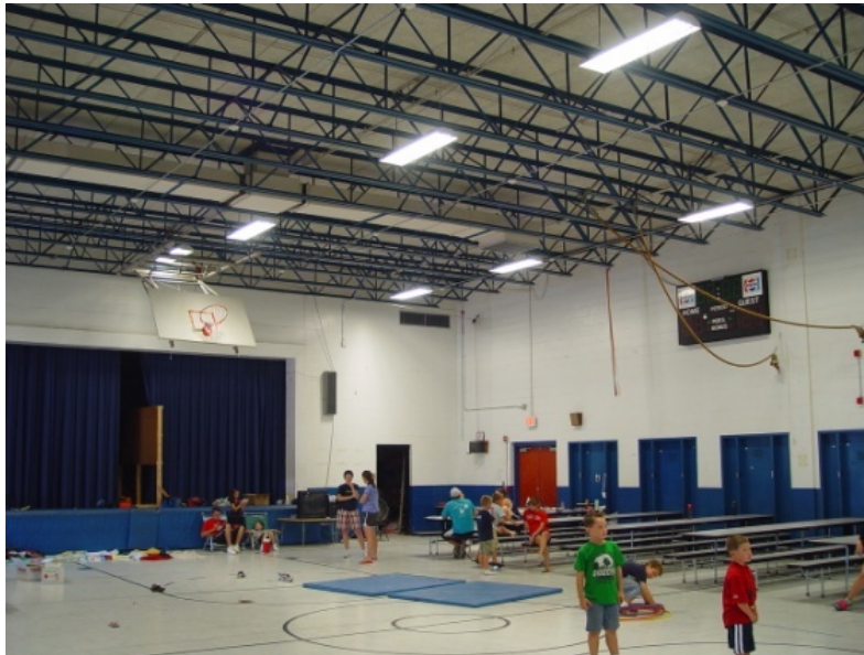
Figure 8. High efficiency lighting in the old gymnasium
