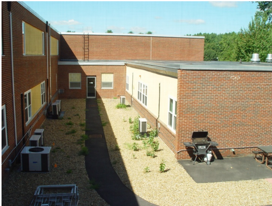
Figure 4. Municipal Building infill panels and ductless air conditioning condensers
