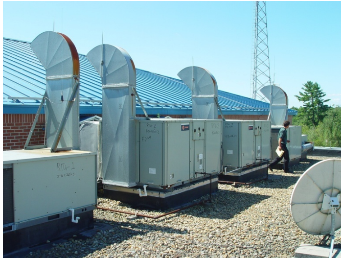
Figure 12. Roof top heating, cooling, and ventilation equipment
