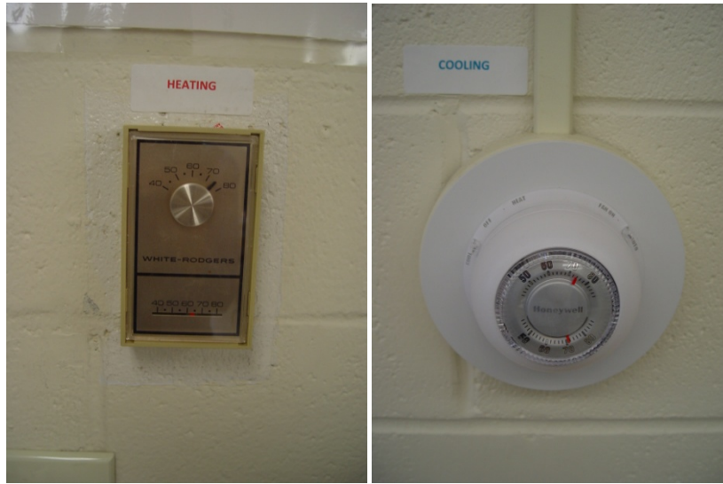
Figure 6. Separate heat and cool thermostats
