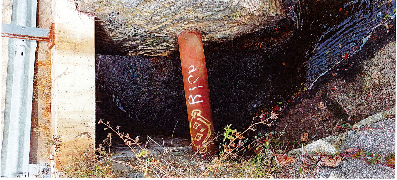
8 Sewer Main Through Existing Culvert
