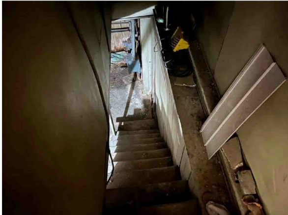
Staircase to Basement
