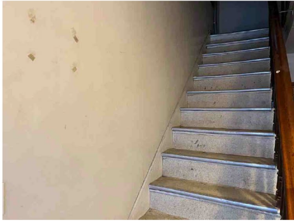
Staircase to 2nd Floor
