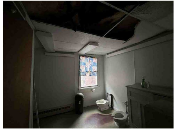
Interior of 2nd Floor
