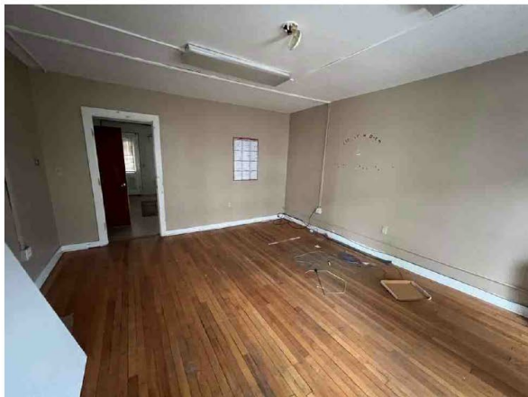
Interior of 2nd Floor
