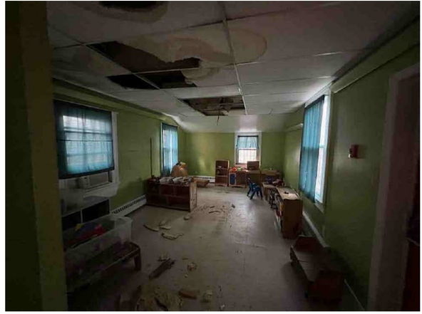
Interior of 2nd Floor
