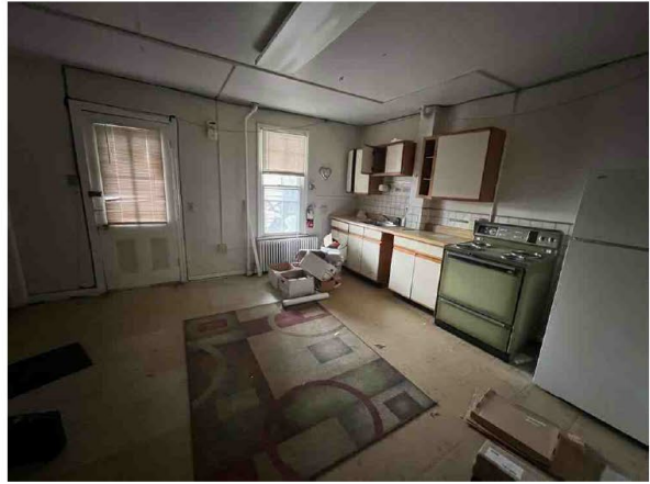
Interior of 2nd Floor
