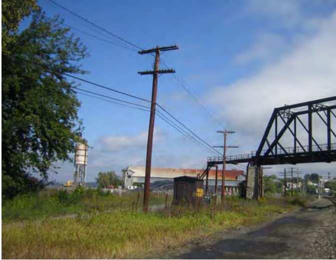
15. Bridge Structure over Railroad
