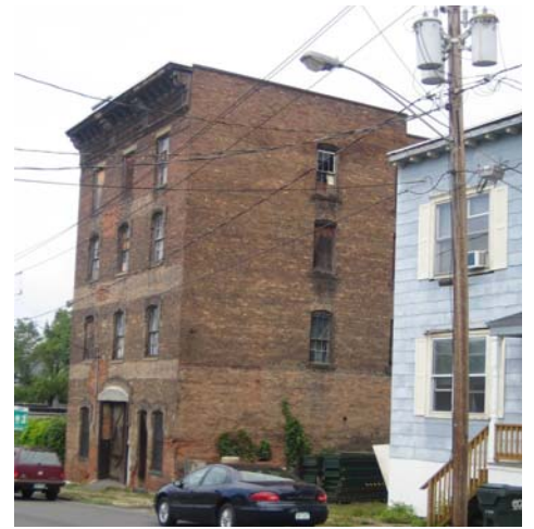
Cobra-style lighting attached to utility poles is out of scale with Hudson's street architecture
