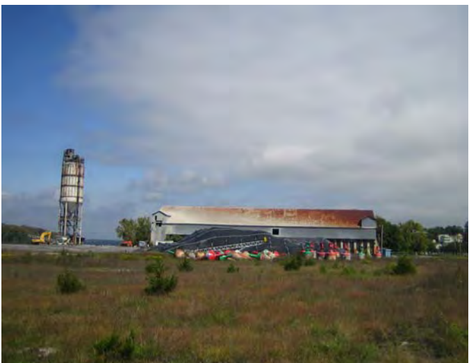
5. Holcim Port Property
