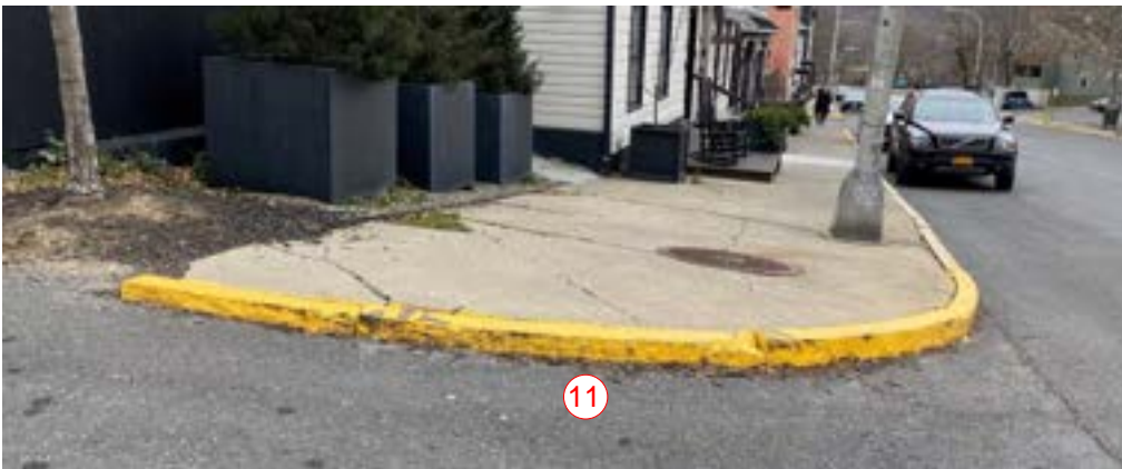
Photo Reference J 11 - Absent curb ramp
