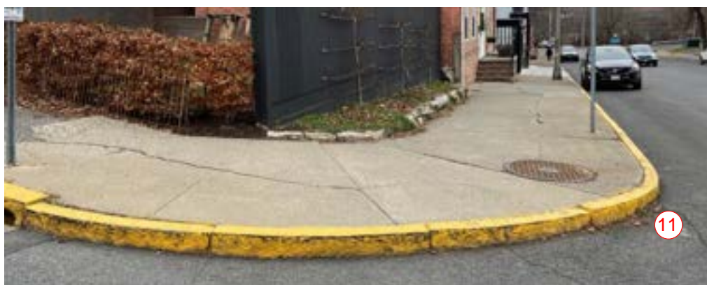
Photo Reference H 11 - Absent curb ramp
