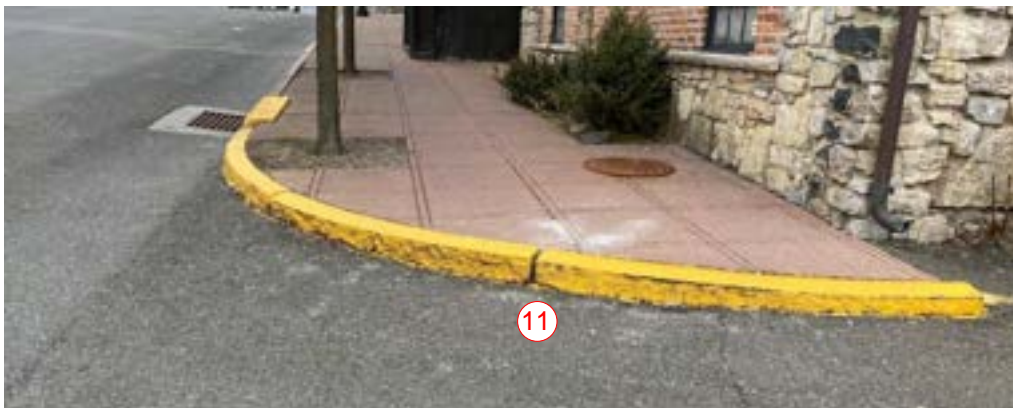
Photo Reference K 11 - Absent curb ramp
