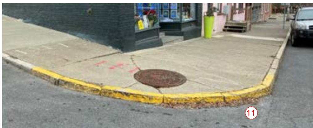
Photo Reference F 11 - Absent curb ramp
