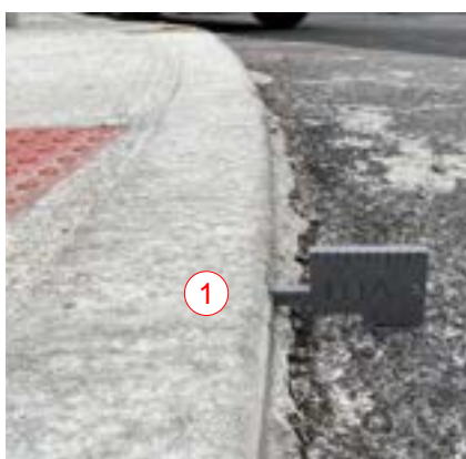
Photo Reference G 1 - Greater than 1/4" level change at ground surface
