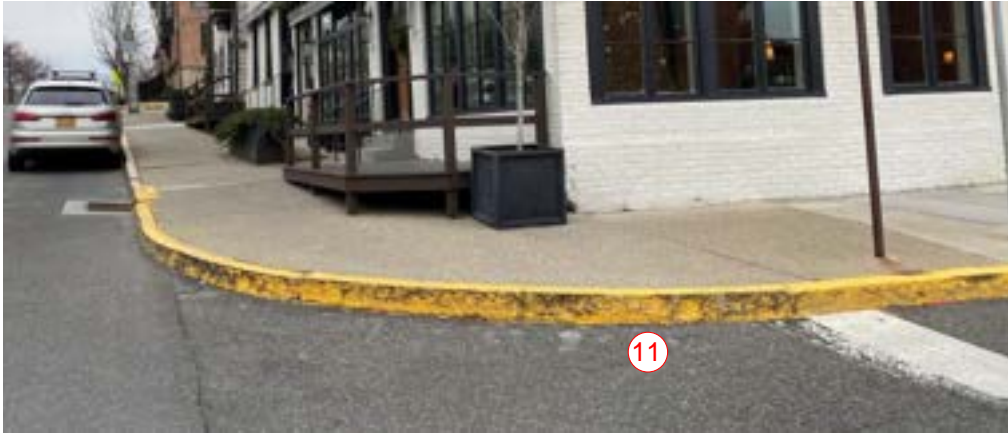
Photo Reference I 11 - Absent curb ramp
