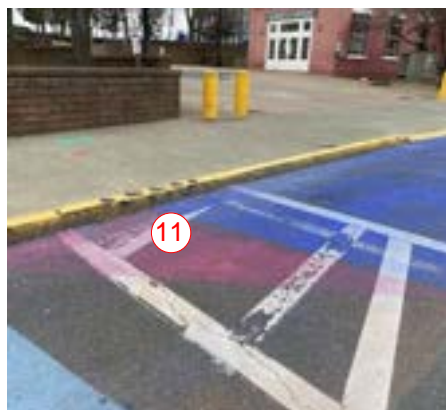
Photo Reference L 11 - Absent curb ramp
