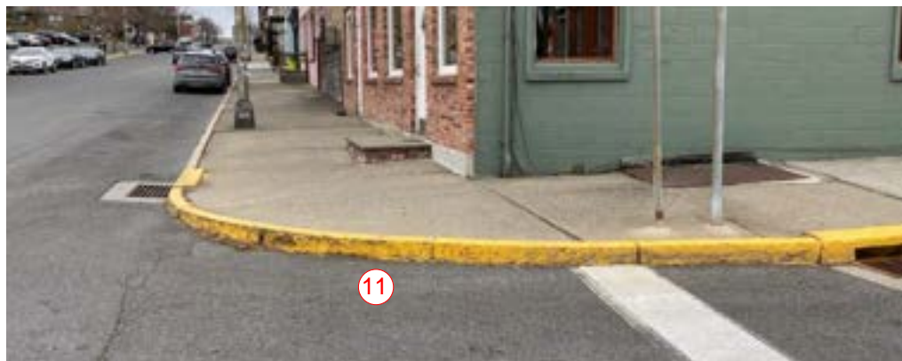
Photo Reference E 11 - Absent curb ramp
