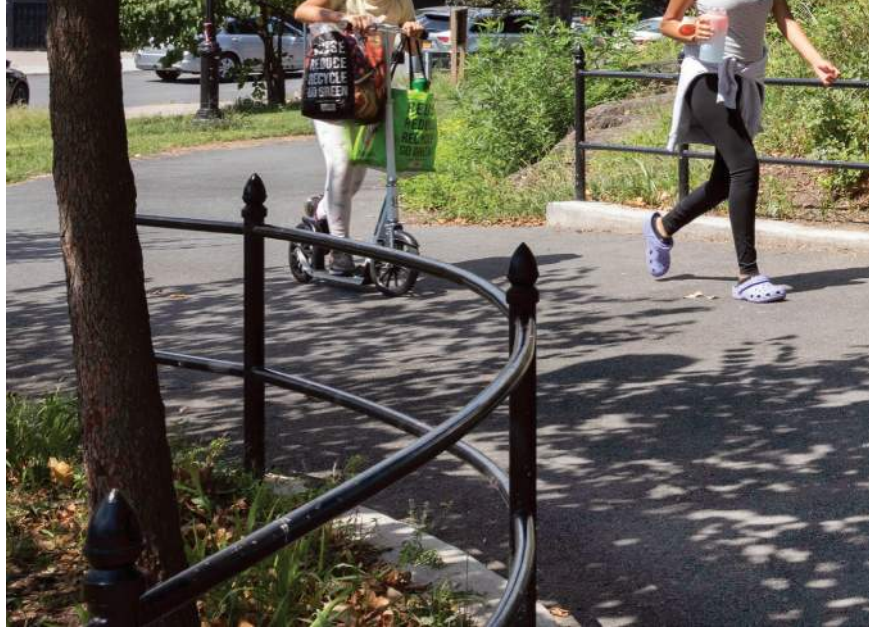
PIPE RAIL FENCE
