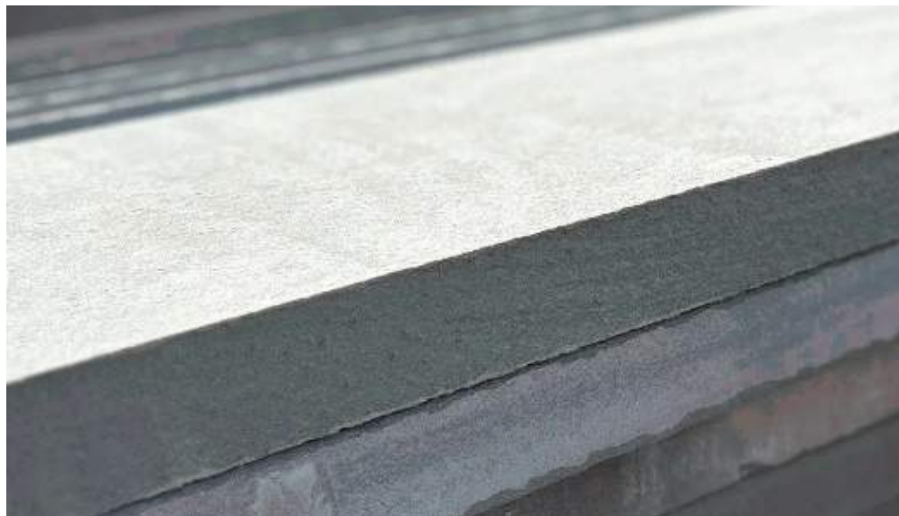
BLUESTONE CURB - 4" WIDE FLUSH BORDER TO PATH
