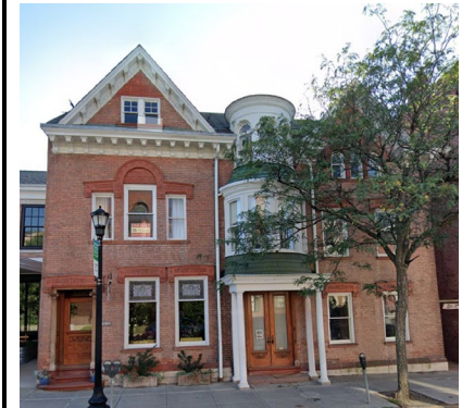
445-447 Warren Street (dated photo; green roofing is presently grey monotone synthetic slate)
