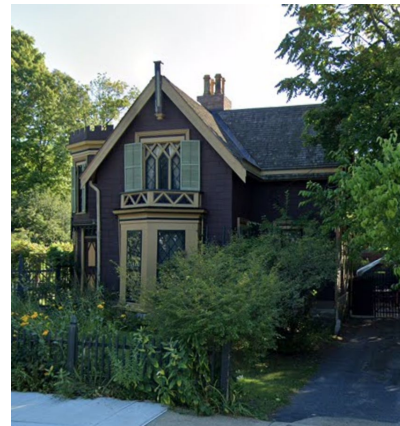
611 Union Street (example of synthetic shingle roofing)
