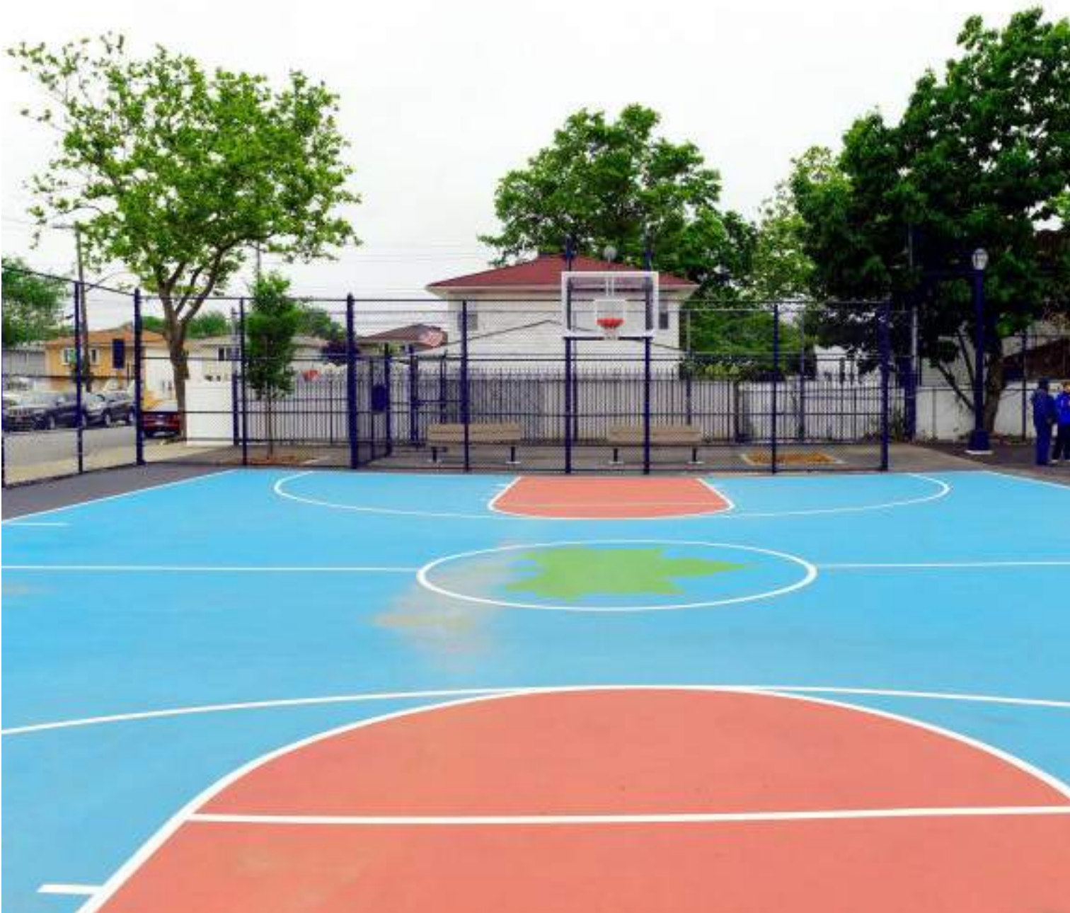
New basketball court with color seal coat, 12’ height fence at either end, pvc coated chain link
