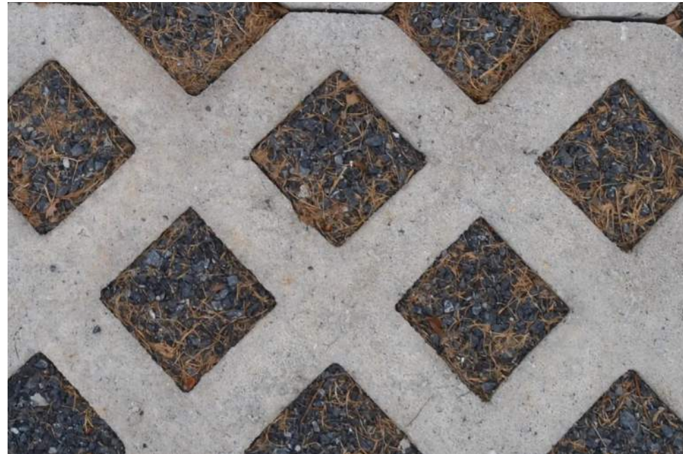
Permeable pre-cast pavers.
