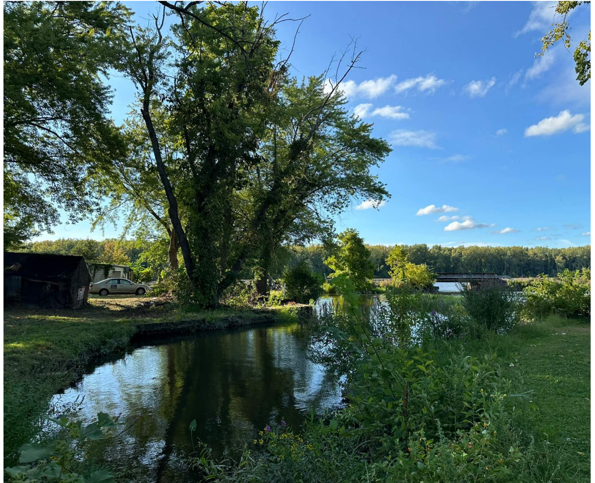
Boat launch with timber bulkhead and existing shacks beyond, August 2024.
