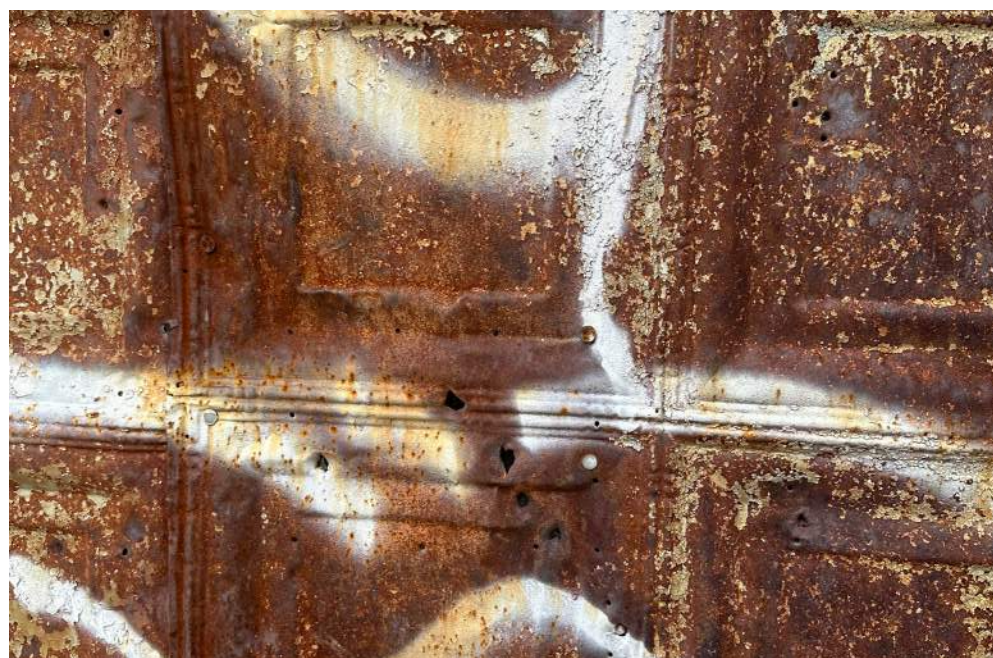
Shack siding material enlargements. Prior to demolition, materials should be cataloged and historically significant components excised and stored for potential future reconstruction or exhibition.
