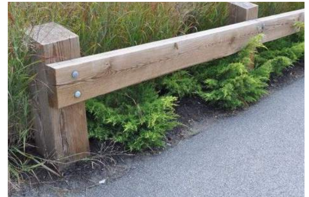
Timber rail to control vehicles.
