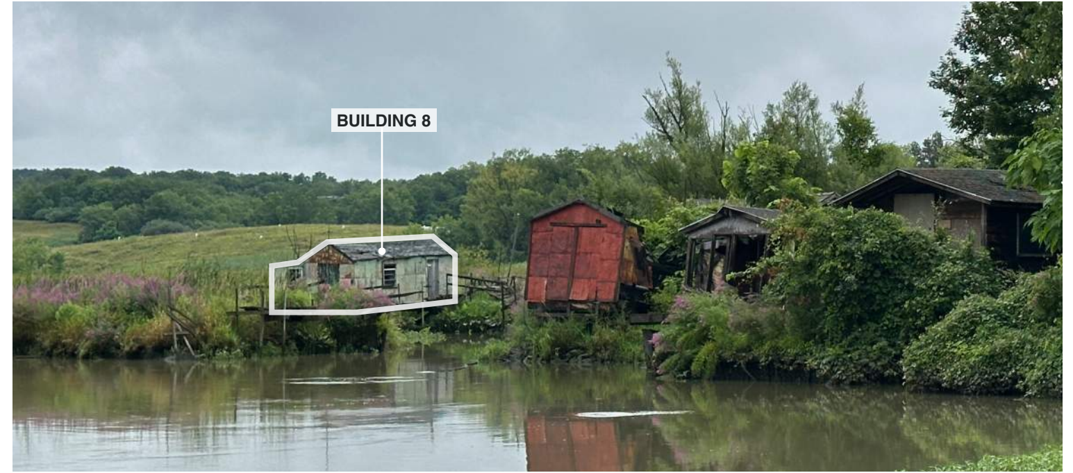
B. SHPO recommends Building 8 be mothballed.
