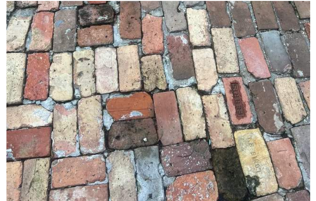
Recycled brick or cobble pavers.
