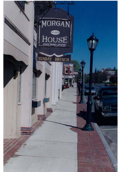
Use of pavers along concrete sidewalk, accommodating street lighting
