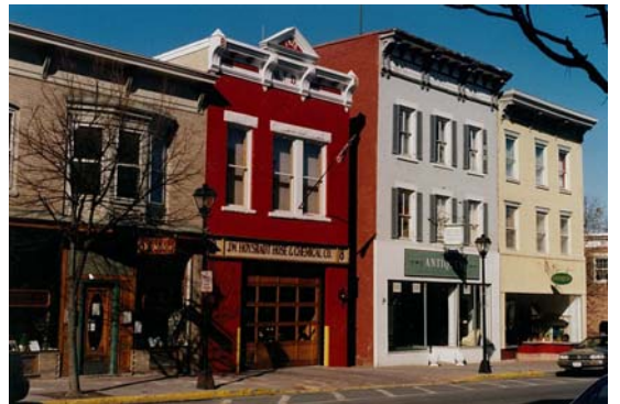
Simply designed signs relate to building facades along Warren Street
