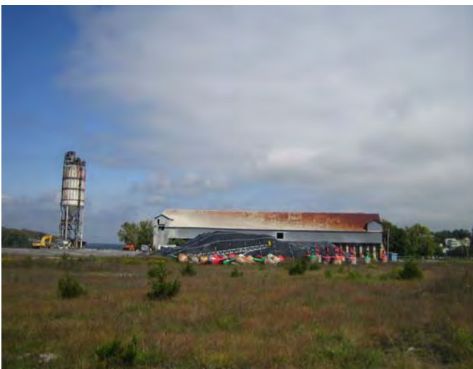
5. Holcim Port Property
