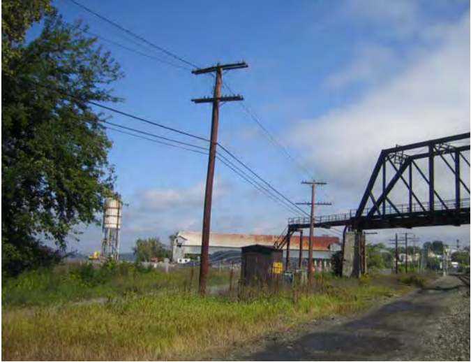
15. Bridge Structure over Railroad
