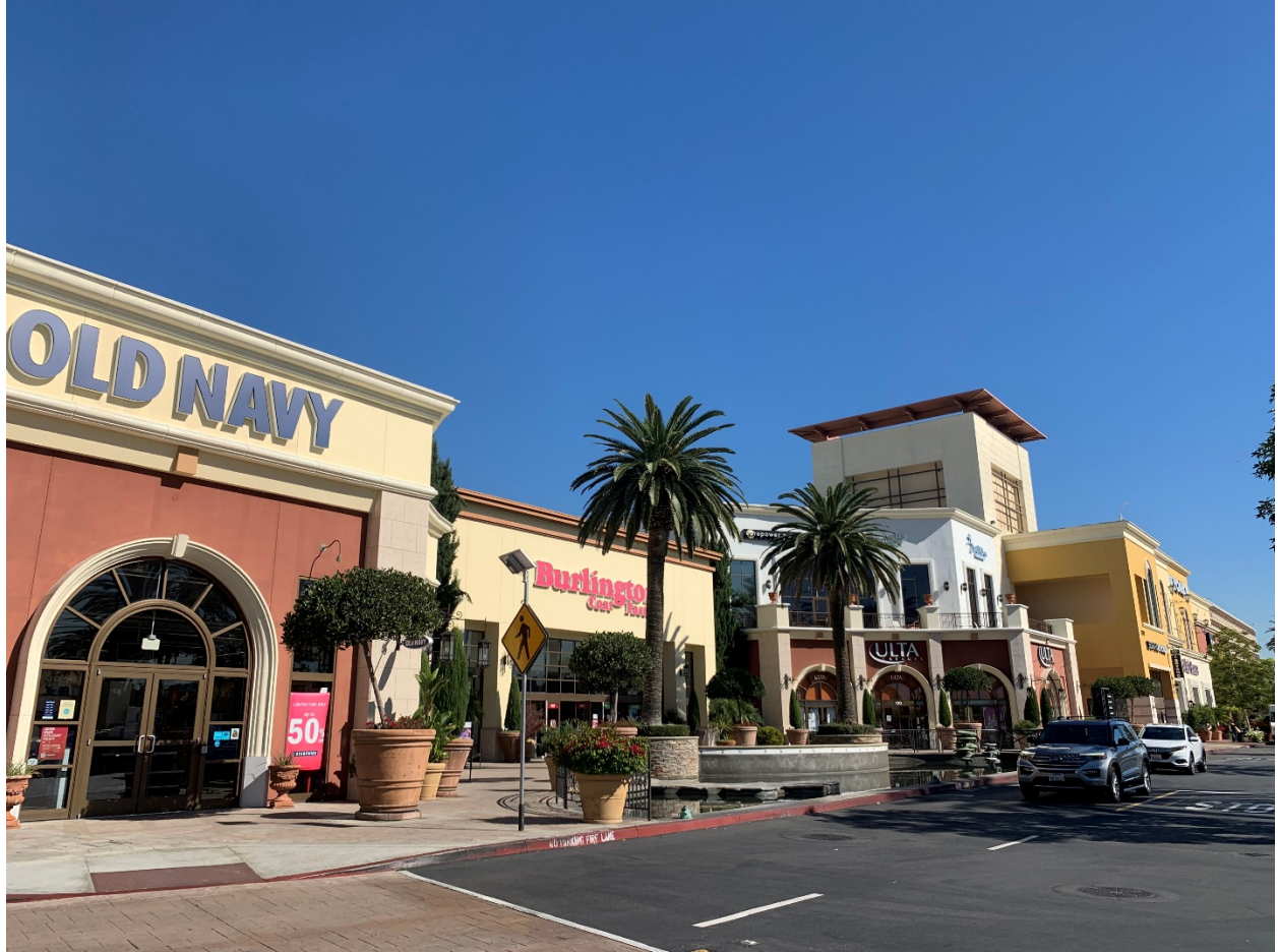
Picture 3: Looking east/northeast along the south (Edinger Avenue) façade (October 2021).
