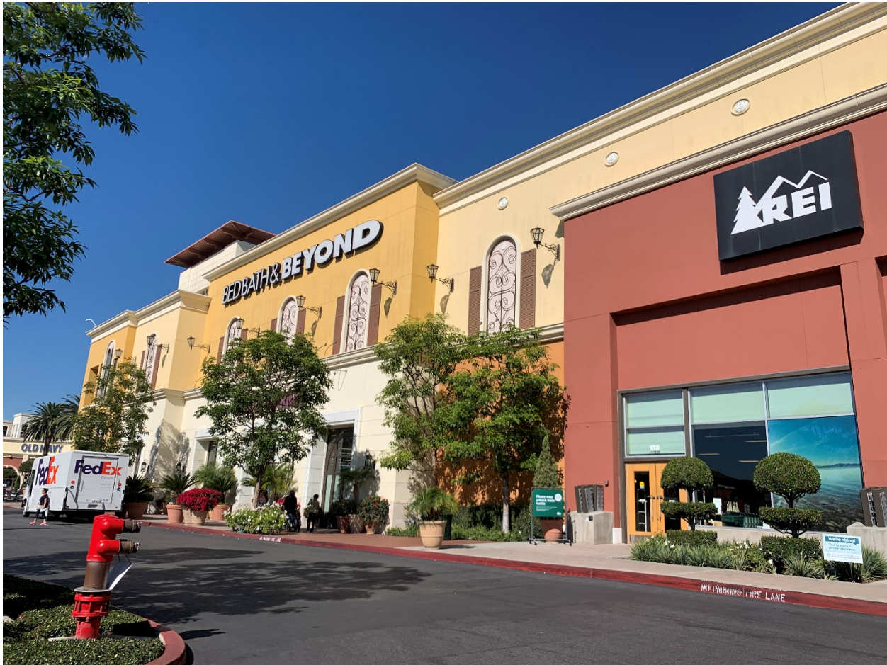
Picture 2: Looking west/northwest along the south (Edinger Avenue) façade (October 2021). This façade style likely dates to the redesign of the mall between 1999-2006.
