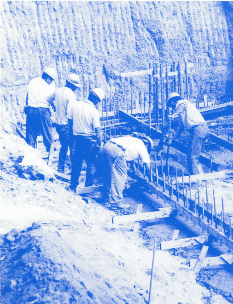
Workmen pour concrete into forms for basement of development building. Altogether, nearly 20,000 cubic yards of concrete were poured into special forms to complete shells of the buildings.
