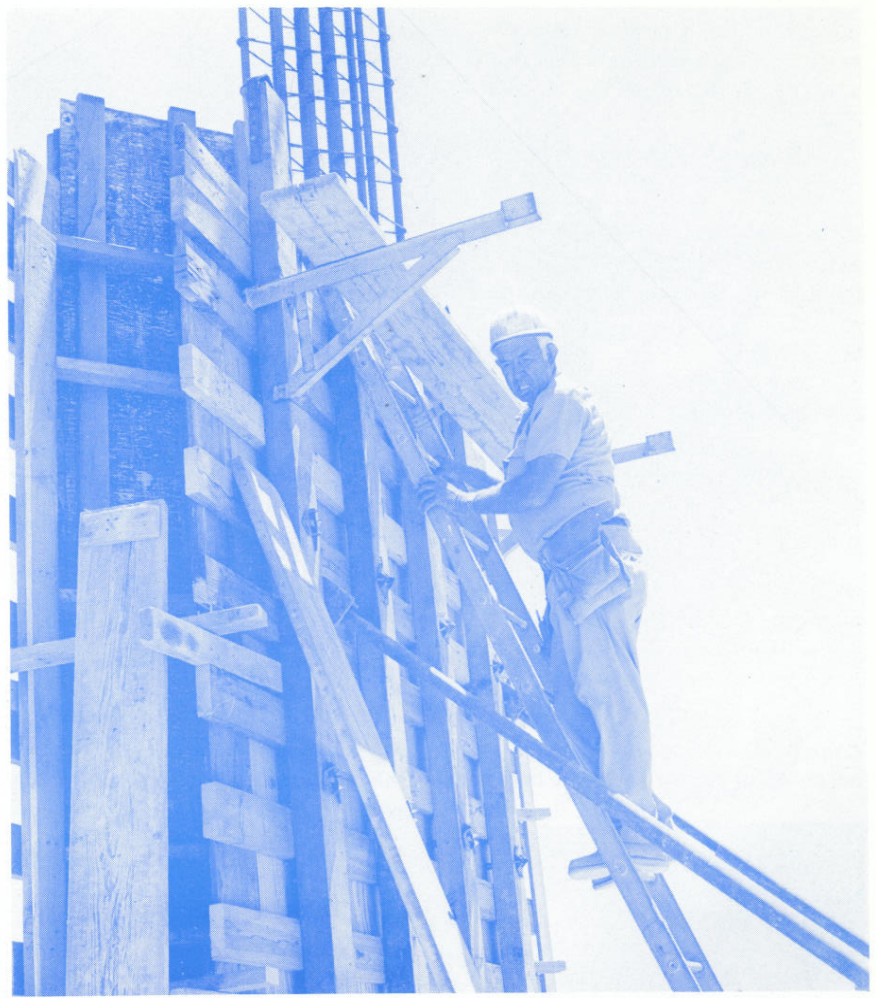
Architect Meyer and the builders of the civic center designed special forms for concrete pouring which would result in maximum progress in construction at a minimum cost. Here a builder is ready to take the forms and the buildings higher. Below, concrete trucks pour walls of the police facility while workmen in the foreground smooth walls already completed.
