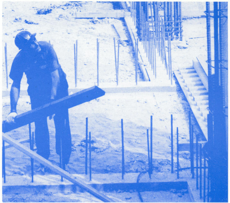
This worker shows an intensity of purpose which resulted in the completion of this $12 million center in the least amount of time with the least amount of troubles. Although there is concrete and steel for all to see, the sweat of man's labor is what will make this building project stand over the decades.
