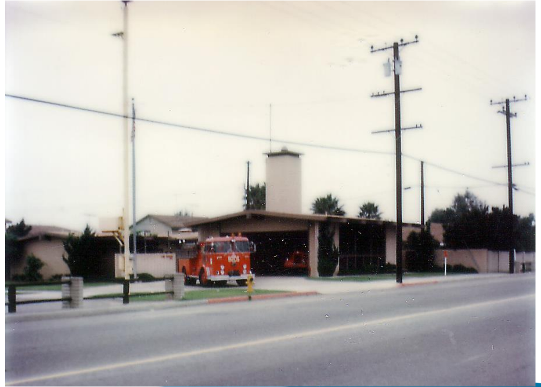
Fire Station 3 – Bushard - (1976)
