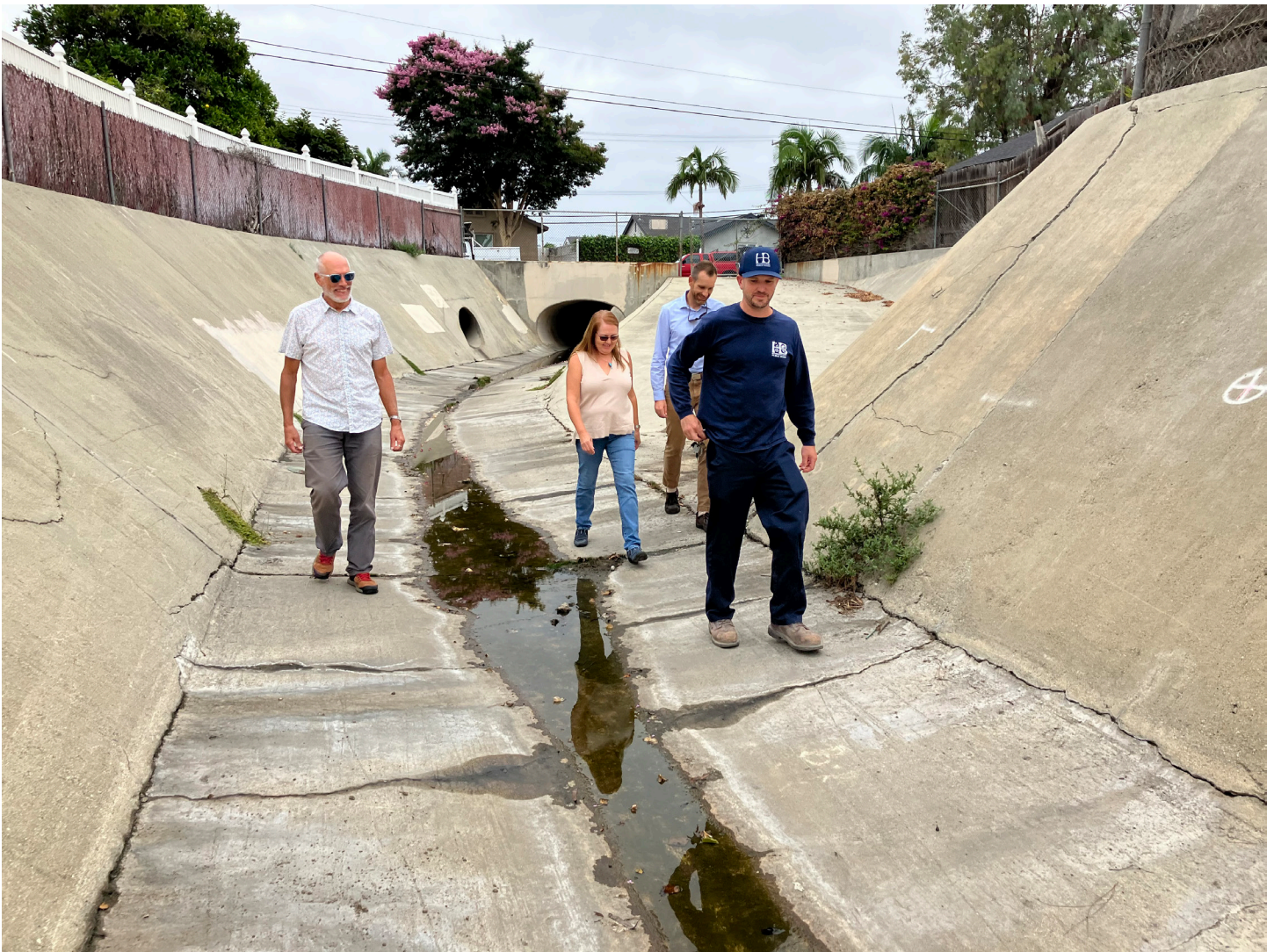
A tour inspects stormwater management systems
