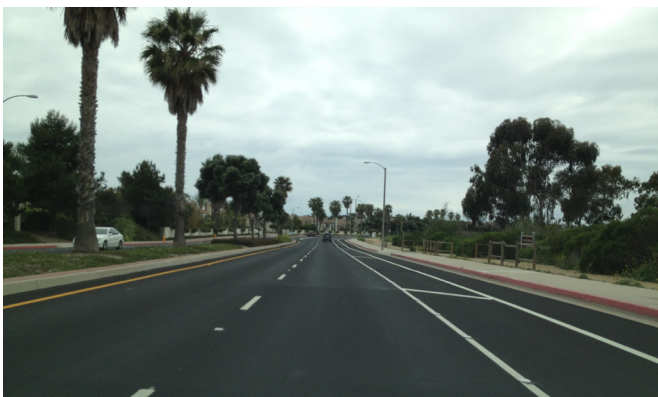
Buffered bicycle lane - Seapoint Drive
