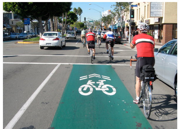
4B) Shared lane markings or "Sharrows" remind vehicle drivers that cyclists can be expected in the roadway and to help cyclists properly place themselves within the roadway. On high bicycle volume streets, a green stripe can be included to further provide horizontal bicycle placement - Oceanside and Long Beach, CA
