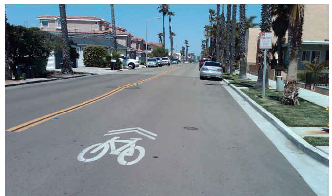
Shared lane marking - Oceanside, CA
