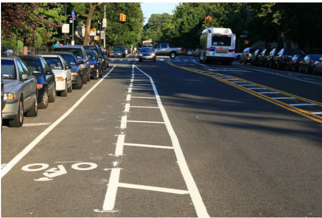
6B) A buffer removes extra space from a travel lane and increases the distance between vehicular and motor traffic. If the extra space is added to the bicycle lane and not diagonally striped, the bicycle lane can appear wide enough to be confused with a travel lane - Top: Huntington Beach, CA (Photo credit bottom: APBP)
