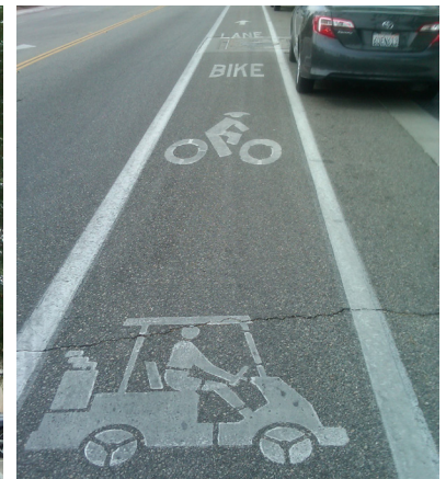
Shared lane signage and markings - Palm Desert, CA (Source: Alexander Meyerhoff, City Manager, City of Holtville)
