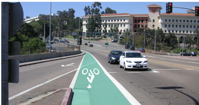
Green transition lane (Simulation) - San Diego, CA
