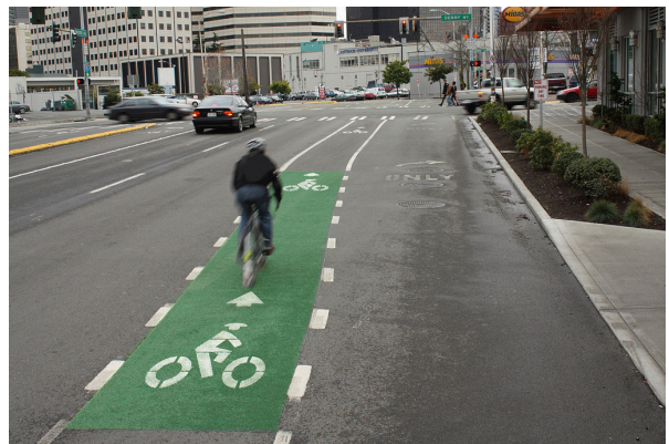
9B) Color in the bicycle lane is a visible reminder to vehicle drivers to expect cyclists in the bicycle lane (Photo credit: Seattle DOT)
